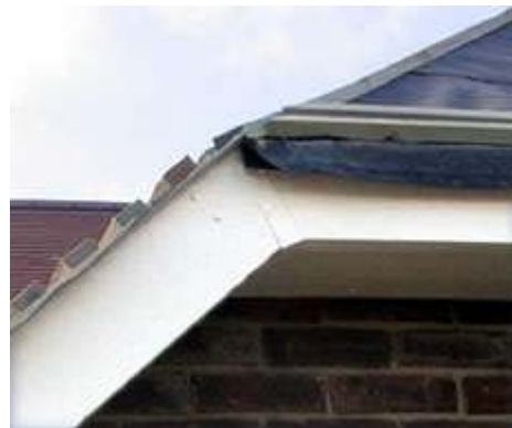
Eaves end and bargeboard on part-hipped roof
