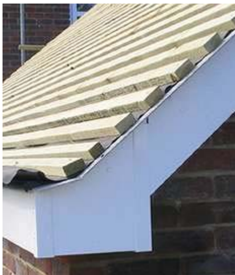
Eaves end and bargeboard on part-hipped roof
