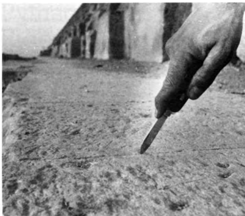
Casing blocks of the Great Pyramid of Cheops. Made of dressed white limestone cut to tolerances that today could not be equalled easily or economically, or perhaps at all. The point of the penknife cannot be inserted between two blocks. In the interior of the temple, blocks as finely dressed as this weigh up to 10 tons.
