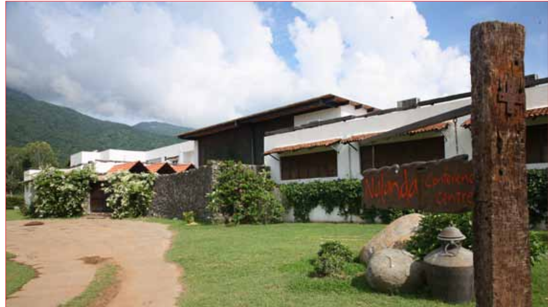
Nalanda Conference Center located at the Isha Yoga Center, Coimbatore is the venue for Inner Engineering Retreats. It also offers modern facilities for exclusive executive meetings combined with yoga and rejuvenation regimes.
