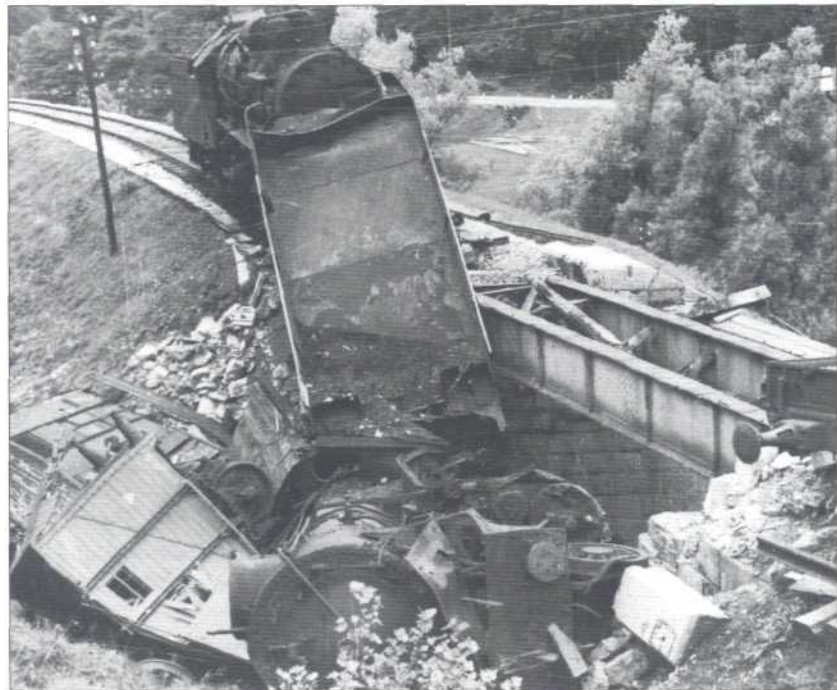
Partisan guerrillas began by sabotaging railways, as shown in this photo. The vital line Zagreb-Belgrade was mined no fewer than 595 times. Explosives were mainly procured from unexploded bombs, artillery shells and field mines.
