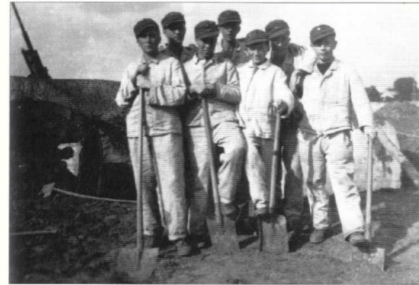
Flakhelfer often spent much of their time on labour tasks, repairing or maintaining their installations. This group, photographed in September 1943, seems to be building a concrete-lined shelter. They wear Luftwaffe fatigue uniforms with their Luftwaffenhelfer caps. (Author's collection)
