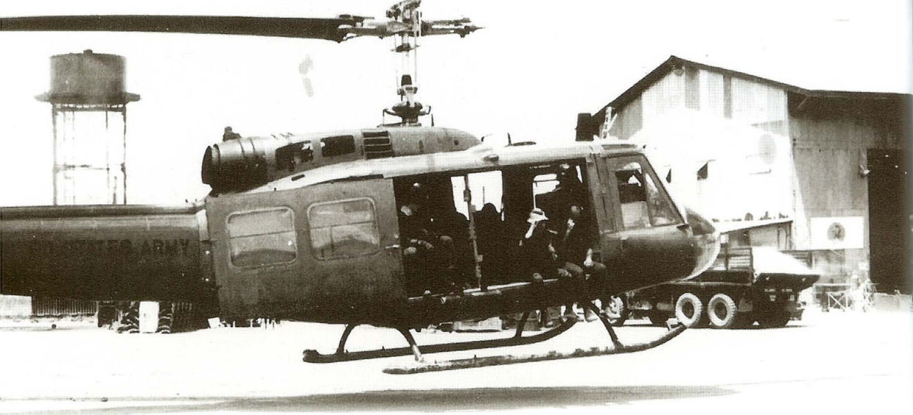
A UH-1H "slick" with the troop compartment doors locked open. It is in ground effect, hovering as it taxis to its takeoff position. (Leroy "Red" Wilson)
