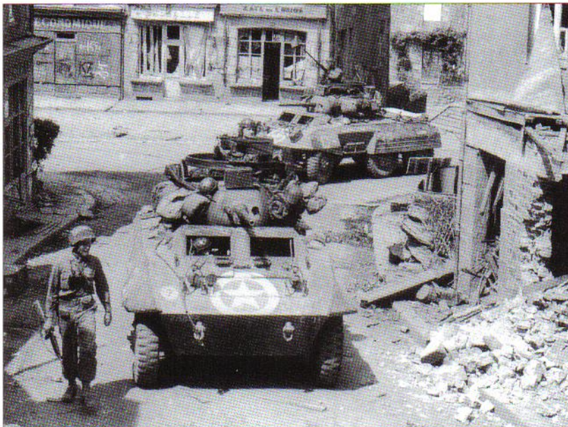
A pair of M8 armored cars of Company C, 82nd Recon Bn., 2nd Armored Division pass through the road junction at St. Sever Calvados on August 3 1944 during Operation Cobra. They have a machine gun ring field mount so commonly seen in Normandy. This unit welded .50-cal. ammunition boxes to the mount, including one box on top of the gun mantlet. The vehicle to the rear, C-32, is from the July 1943 production run. (NARA)
