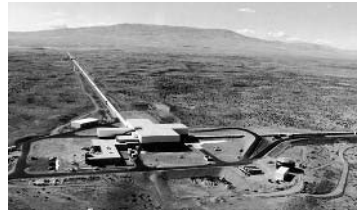
FIGURE 30 LIGO, in Washington State, consists of two 4-km arms at right angles, each with laser beams in high vacuum. There is an identical observatory in Louisiana, and the two installations will work in tandem. The objective will be to detect gravity waves by searching for changes in length a thousand times smaller than an atomic nucleus.
