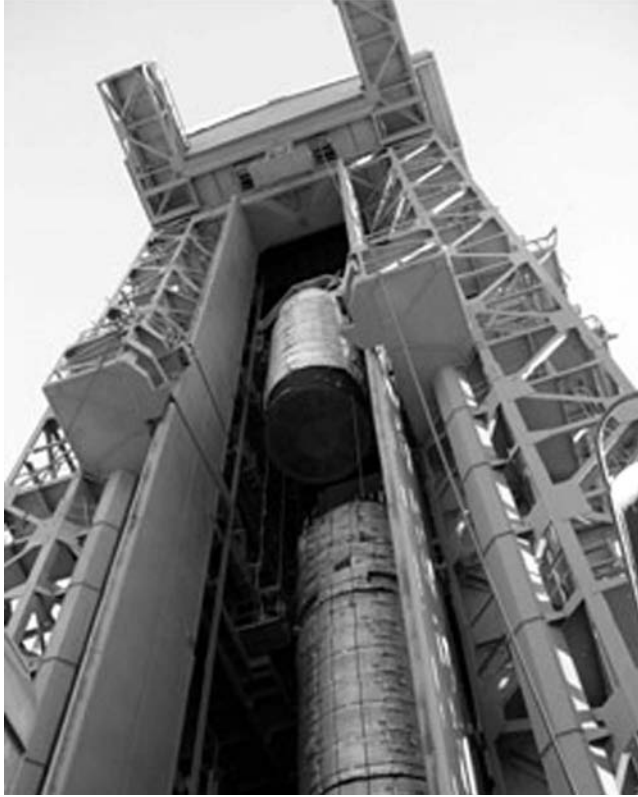
Rockot being raised
