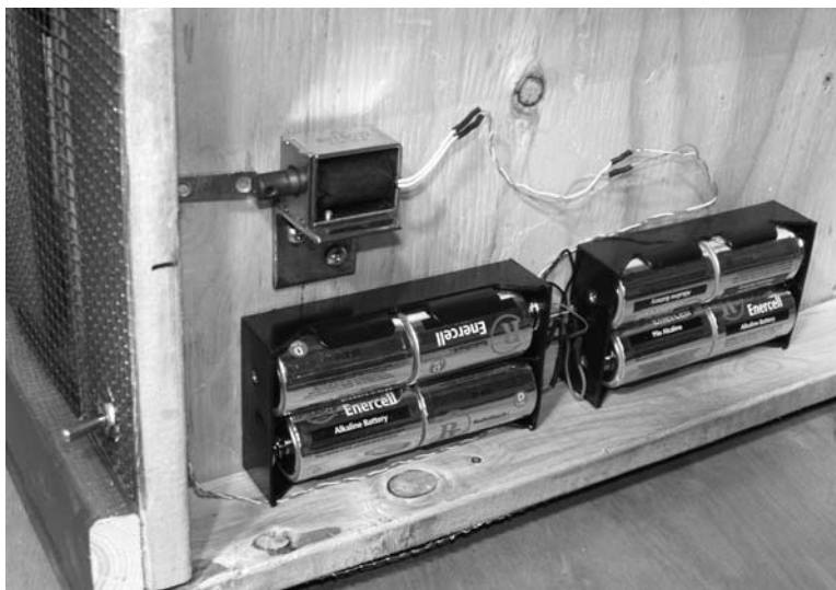
Figure 11-15 Installing the battery packs under the cage
