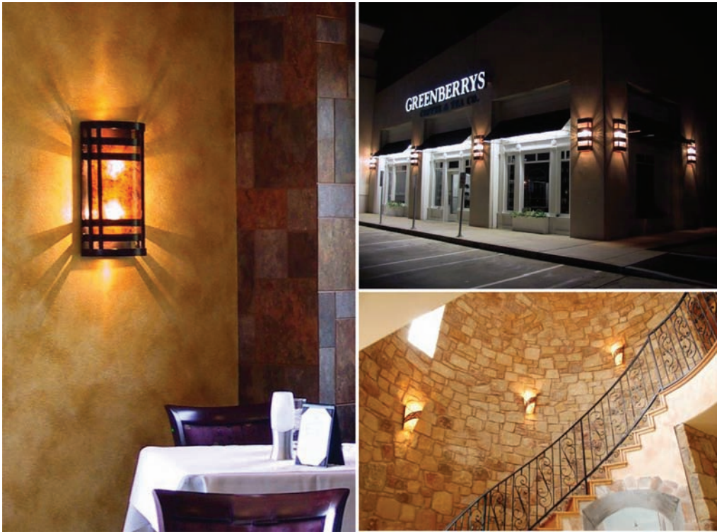
FIGURE 40.4 Wall sconces for providing ambient lighting and the much needed vertical illumination in various situations.
