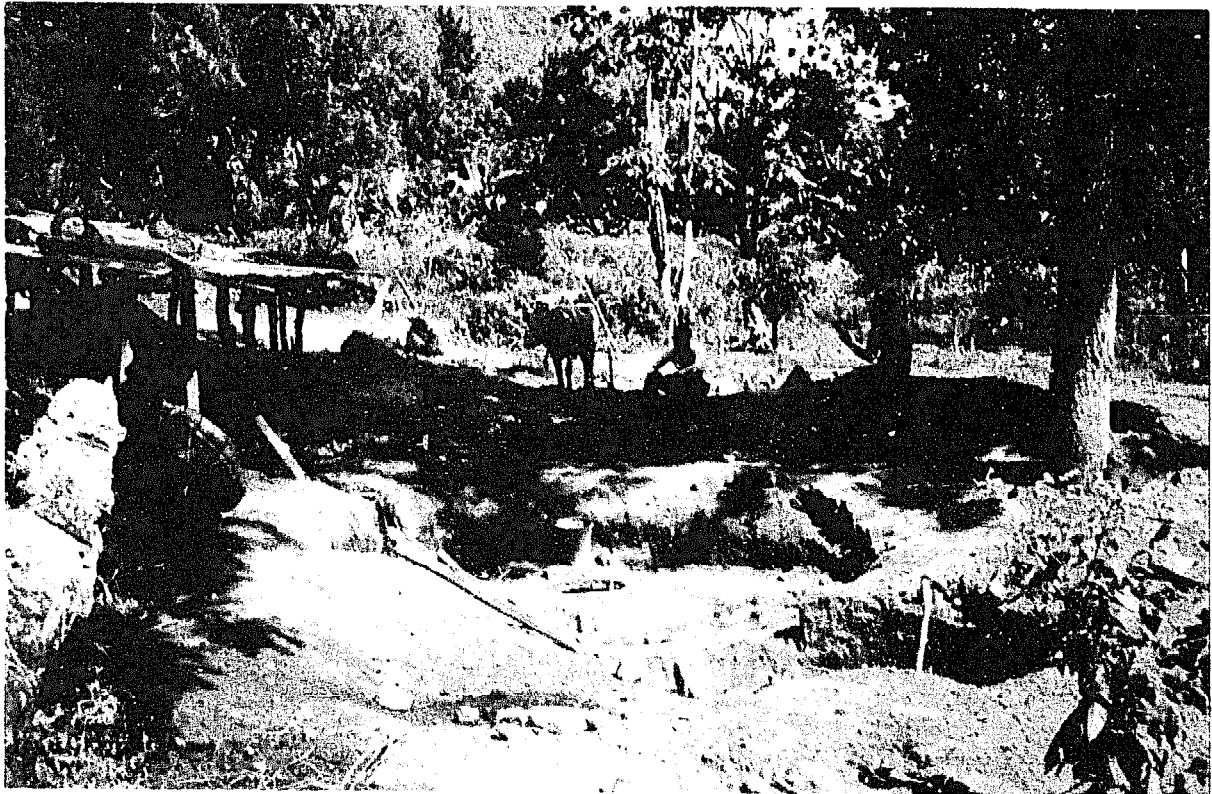
Photo 11: A nearly finished fixed-dome plant in combination with cattle shelter (Source: OEKOTOP, BEP Tanzania)
