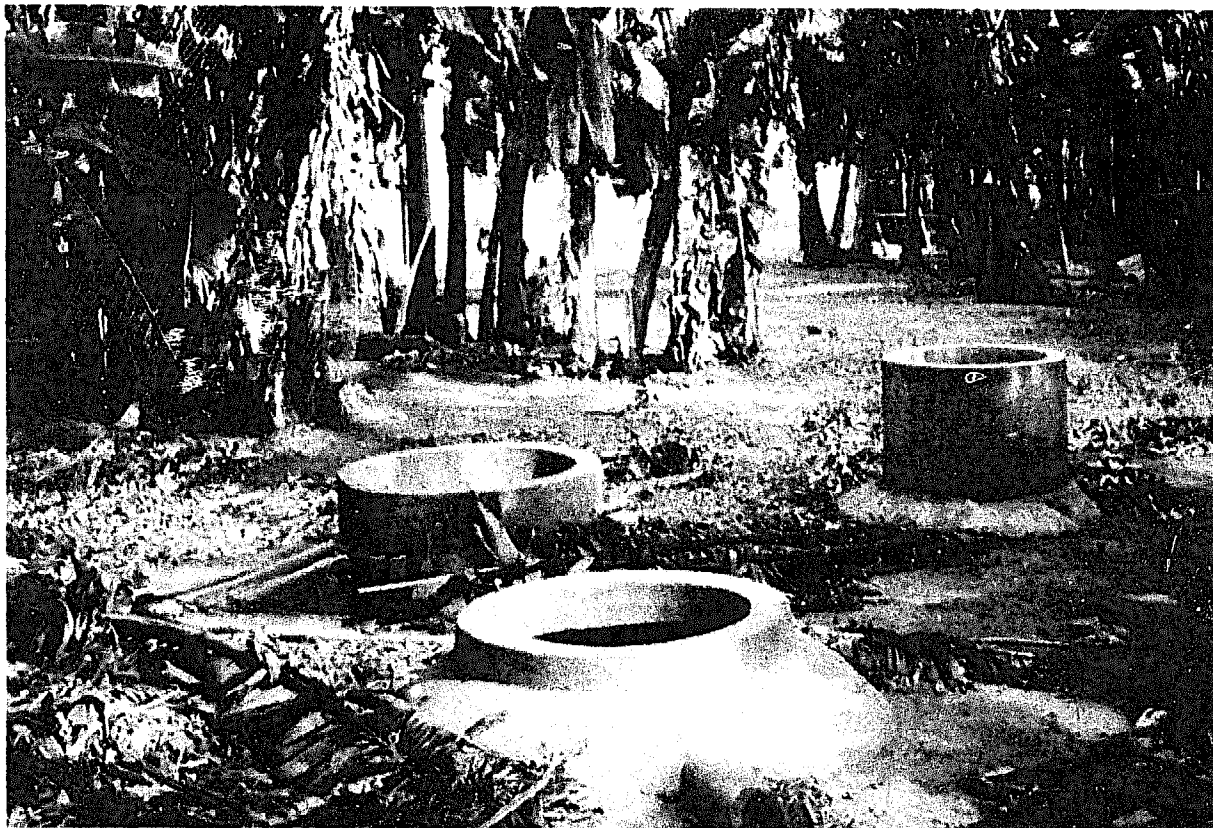
Photo 2: Fixed-dome plant with displacement pit in the foreground, entry hatch at center left, and inlet mixing pit at rear (Source: OEKOTOP)
