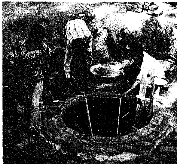
Photo 15: Installing the neck masonry of a fixed-dome (Source: OEKOTOP)
