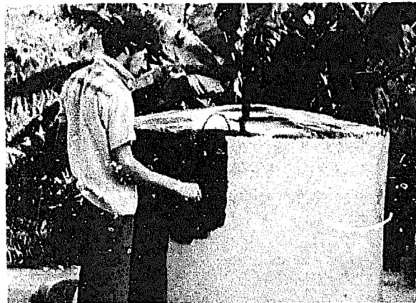
Photo 28: Painting the gasholder (Source: OEKO-TOP/BEP Caribbean)
