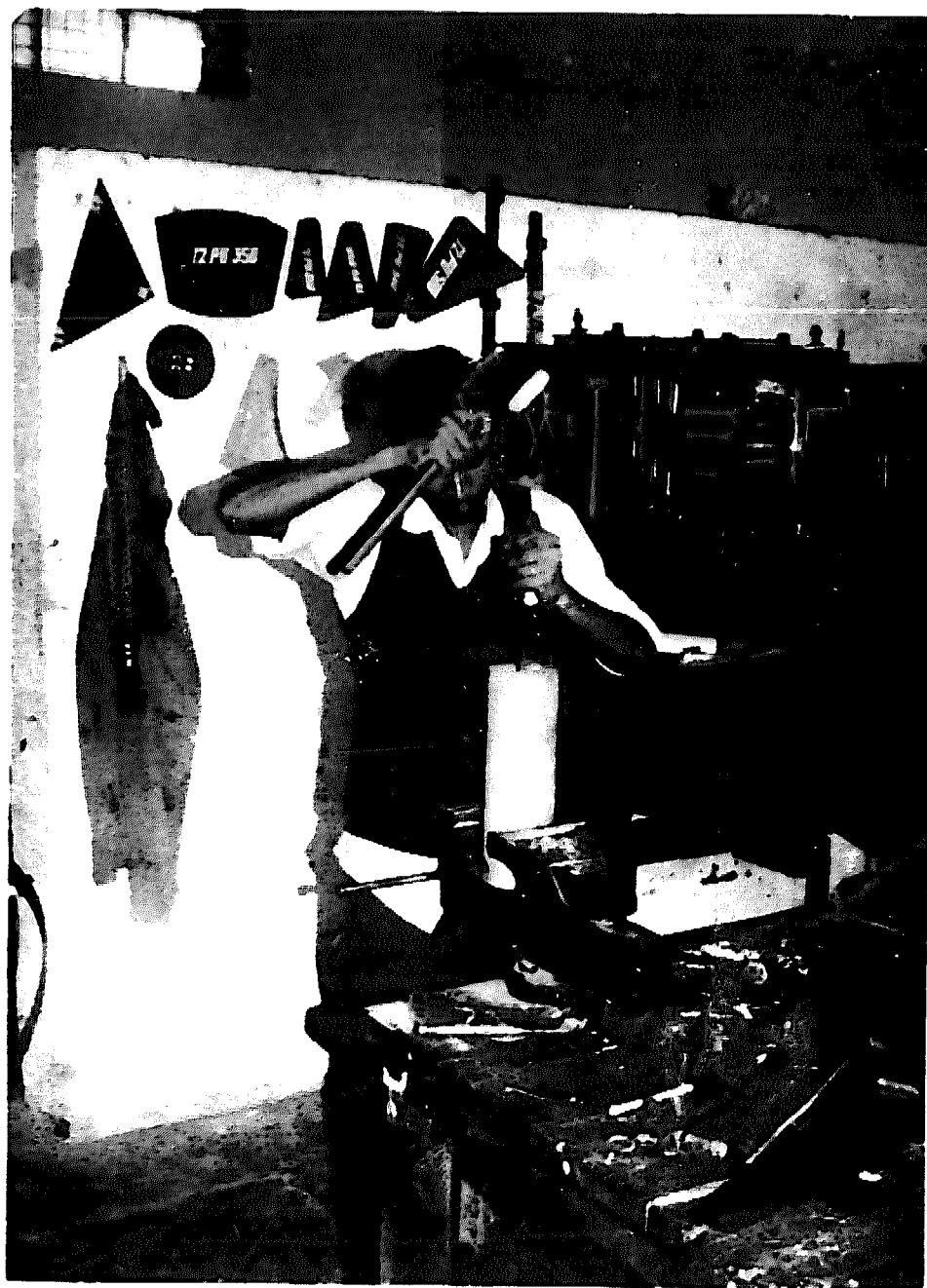
Chiseling the square hole in the crosshead
