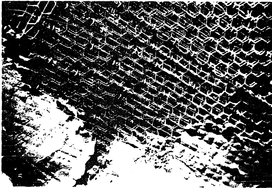
FIGURE 19 Fresh mortar applied to multiple layers of chicken-wire mesh on a 45-foot boat—showing the low-moisture mix that produces a watertight structure. (Noel D. Vietmeyer)
