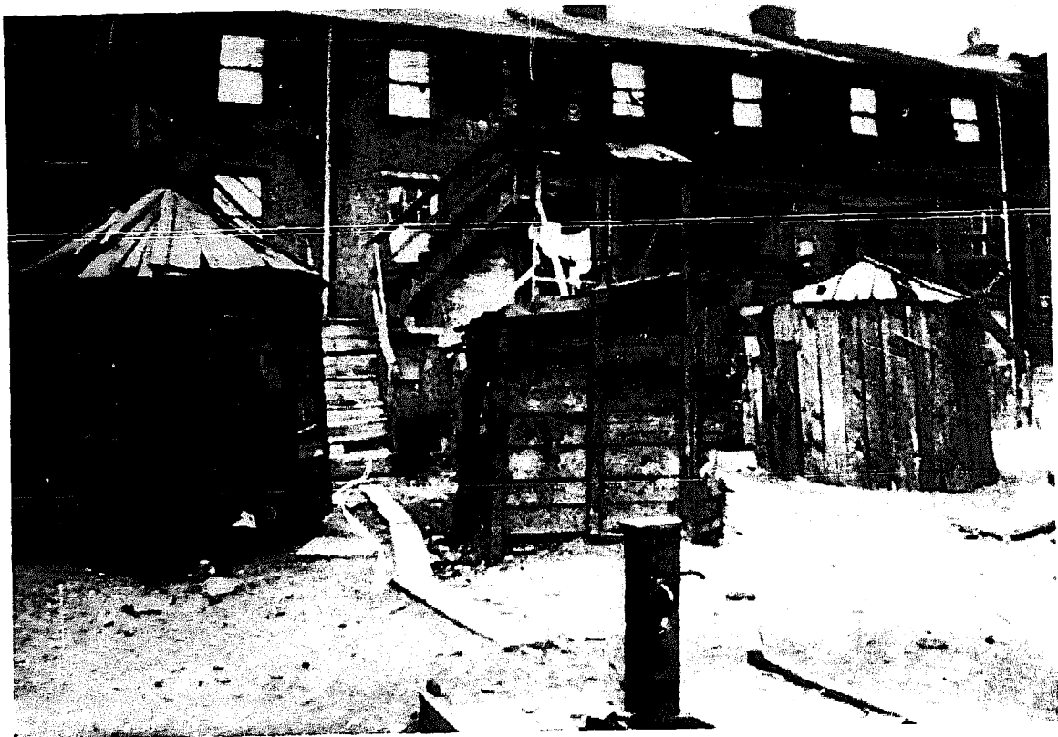
View of backyard in Pittsburgh before the city sewerred up.
