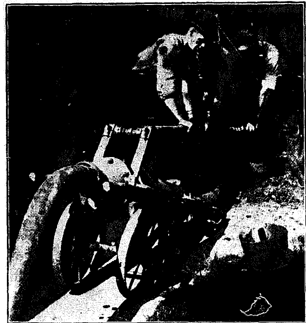
Manually pumping the night soil from privy to tank wagon. (From Survey, September 2, 1911.)
