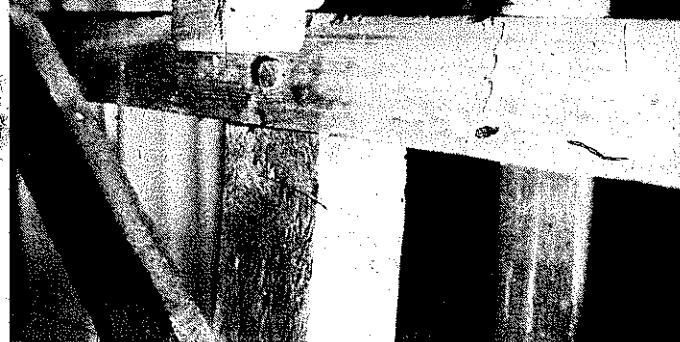
PLATES 261-262 These two photographs show how the frame that holds the heddles (the fifty-two-inch bar) fits down over the top of the loom frame. It is not held in place by anything other than notches.
