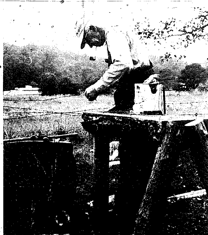
PLATES 320-322. Mr. Dickerson notches the ends of the three legs to fit the battling bench, and then nails them into place. The bench has three legs so that it will set steady, even on rough ground.
