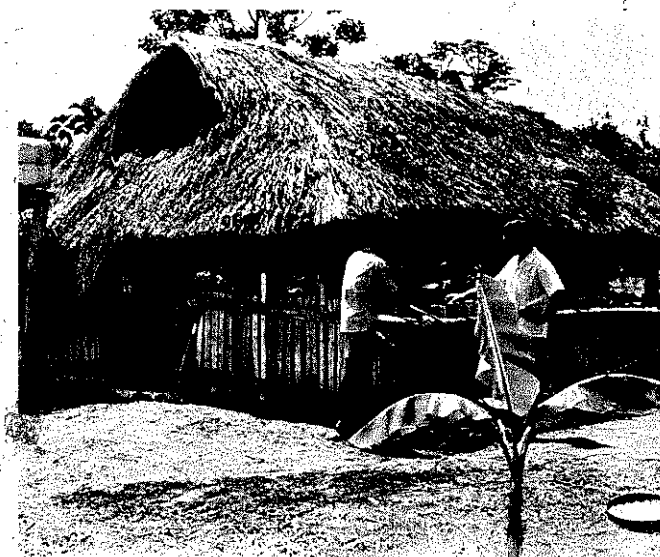
Pig house built of bush materials, Martyrs' High School, NP
