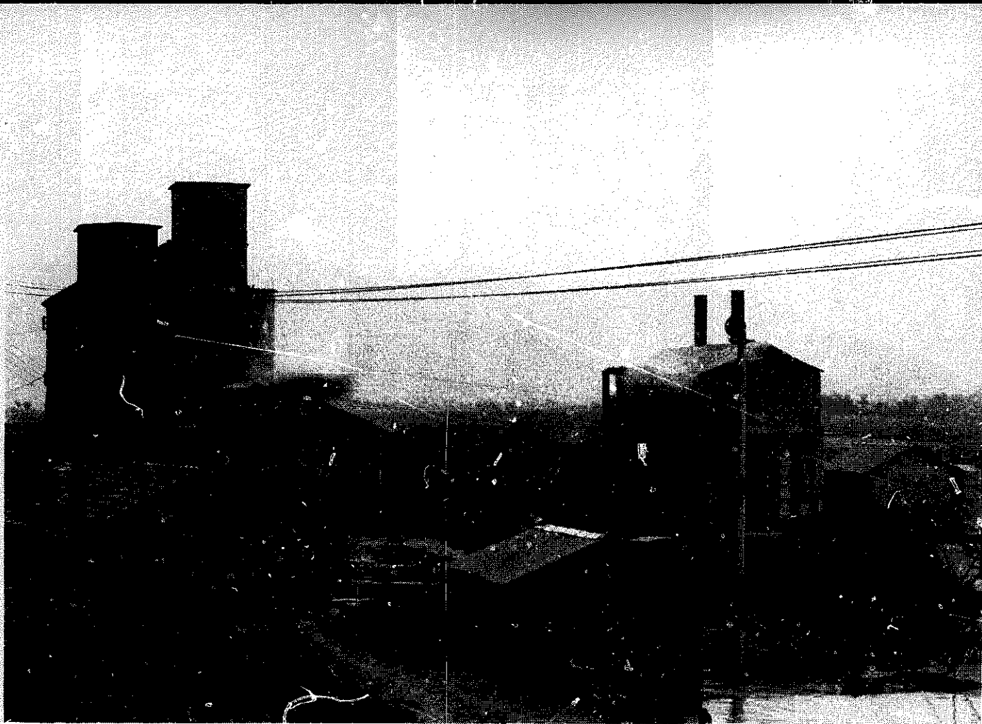
A general view of the plant. The kilns are on the right and the silos are on the left.
