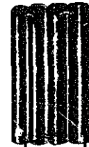
Fig. 7—Shows the two removed, and the four cylindrical tanks connected.
