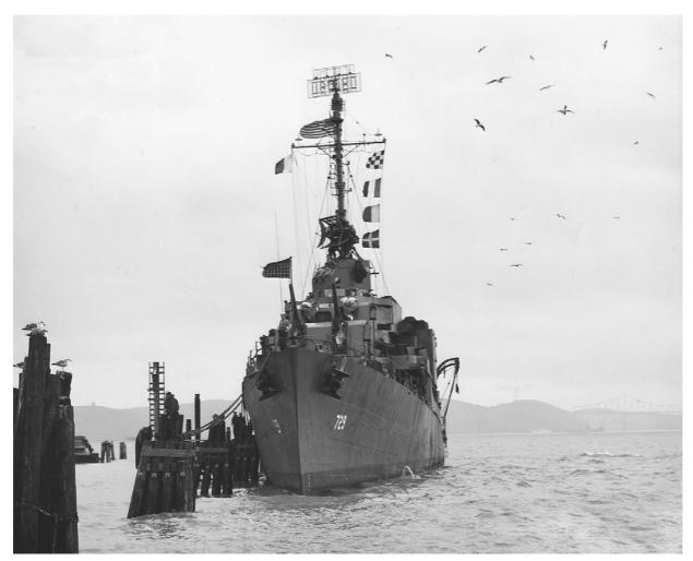
A flaghoist is shown on the USS Lyman K. Swenson tied up off the Mare Island Navy Yard, California, in early 1946. The signal flag on the starboard halliards is "H," meaning "I have a pilot aboard." The four signal flags on the port side are the ship's call letters "NTHR." (U.S. Naval Historical Center)
