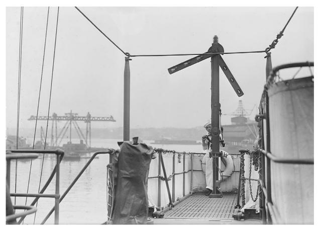
This semaphore signaling device, aboard the battleship USS Utah around 1915, could send ship-to-ship signals across limited distances to supplement flag or radio signals. The horizontal arms could move to represent different letters. (Library of Congress)
