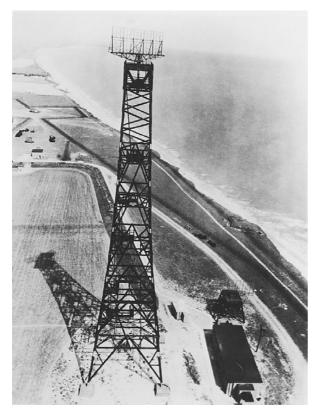
This Chain Home radar antenna, mounted on a 185foot tower, was a central part of the Royal Air Force's technological defense against the German air attack in the Battle of Britain. Multiple similar radar facilities were tied to RAF central command by telephone links enabling rapid fighter defense response to oncoming German aircraft. (Bettmann/Corbis)
