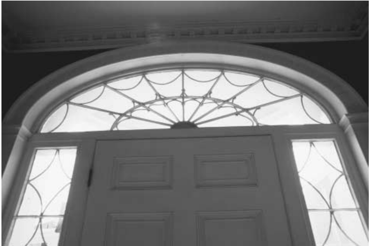
Gardner-Pingree House, Entry. Fanlights and sidelights surround the front door of the Gardner-Pingree House. Such embellishments are characteristic of Federal architecture. © TODD GIPSTEIN/CORBIS.
