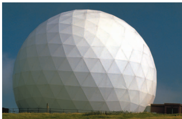
A geodesic radardome at Lowther Hill Civil Aviation Authority Radar Station in Scotland. The dome is made of fiberglass which, unlike concrete, is transparent to radio waves. Photograph by John Heseltine. National Audubon Society Collection/Photo Researchers, Inc. Reproduced by permission.
