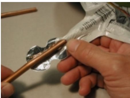
Inserting copper tubing.
