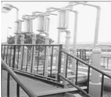
Figure 5.21 (a) Schematic diagram of an airlift pump. (b) Photograph of an airlift pump.
