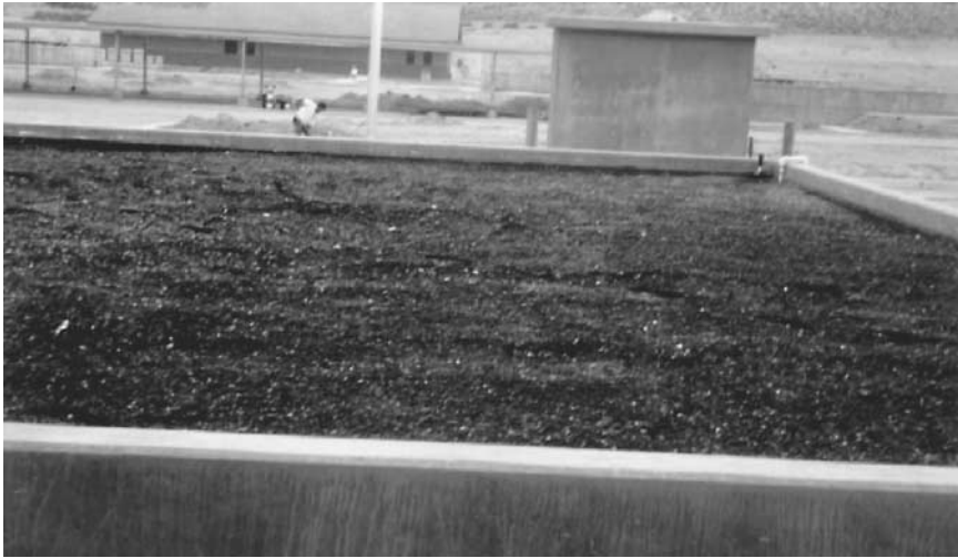
Figure 5.90 Photograph of a soil/compost filter bed used for odor control.
