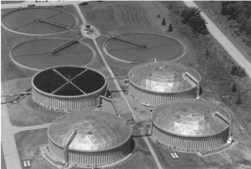
Figure 5.72 Photograph of an aluminum dome covering a trickling filter system. (Courtesy of ULTRAFLOTE Corporation.)
