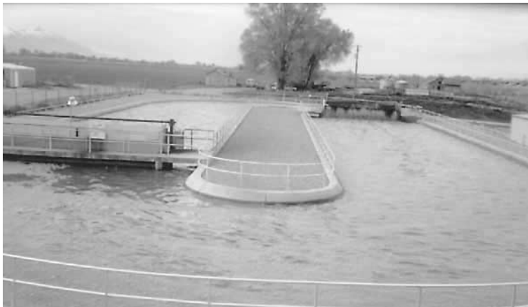
Figure 2.34 An oxidation ditch activated-sludge system.
