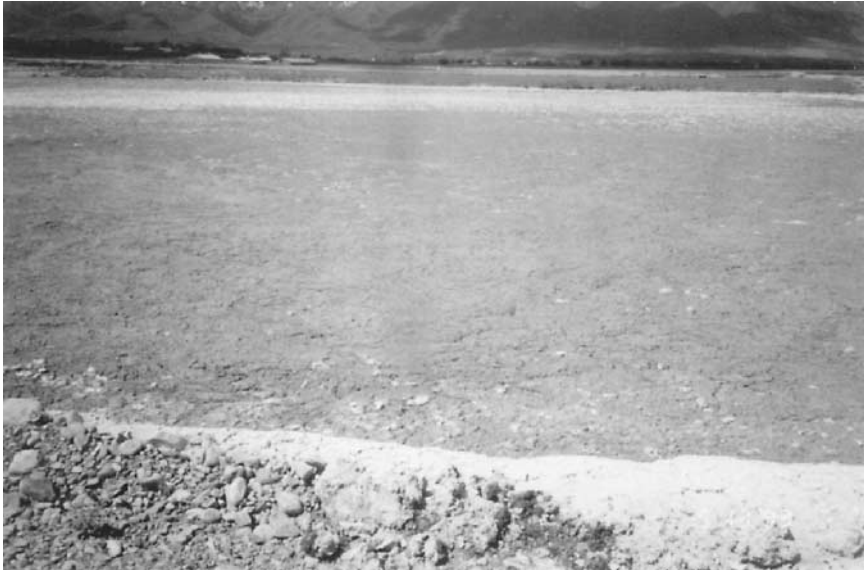
Figure 5.46 Photograph of the scum layer covering an anaerobic liquid sludge lagoon.
