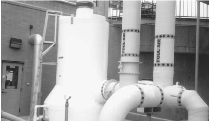
Figure 5.79 Photograph of a full-scale wet scrubber system used for odor control.
