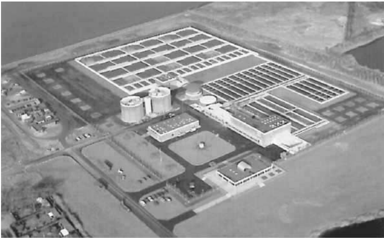
Figure 2.1 (a) Schematic diagram of municipal wastewater treatment facility. (b) Photograph of oxidation ditch wastewater treatment plant. (Courtesy of I. Kruger, Inc.)
