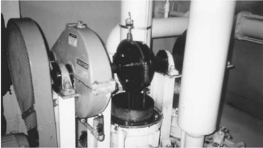
Figure 5.11 Photograph of a plunger pump.
