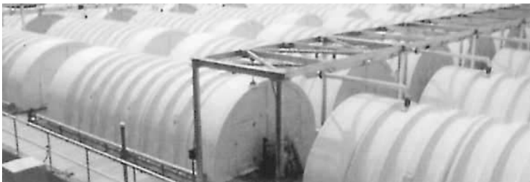
Figure 2.60 A rotating biological contactor system. (Courtesy of US Filter/Envirex Products.)
