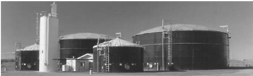
Figure 5.71 Photograph of an aluminum dome covering a sludge storage tank. (Courtesy of AQUASTORE Tanks.)
