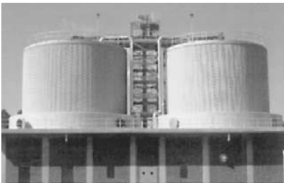
Figure 3.86 (a) Schematic diagram of a vertical tank mechanical compost system. (b) Photograph of a dual-silo mechanical biosolids composting system. (Courtesy of US Filter / Davis Process.)
