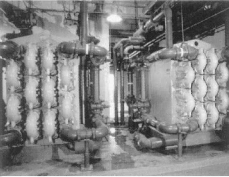
Figure 3.31 A tube-in-tube heat exchanger. (Courtesy of US Filter/Envirex.)
