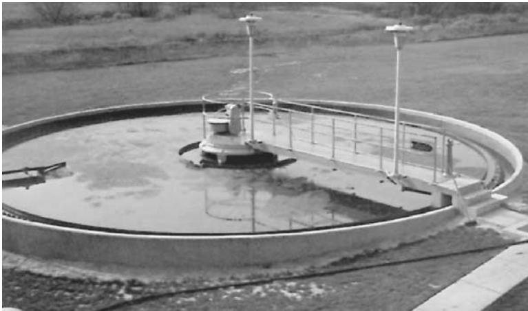
Figure 3.2 (a) Schematic diagram of a gravity thickener. (Courtesy of EIMCO Process Equipment Company.) (b) Sludge gravity thickener. (Courtesy of Dorr Oliver.)
