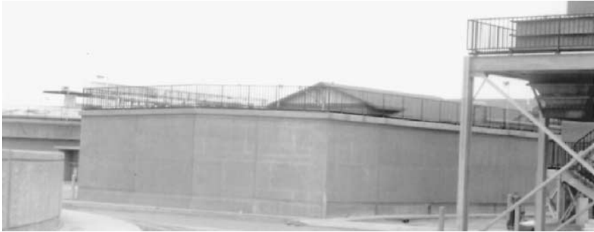
Figure 5.38 Photograph of a sludge holding tank.
