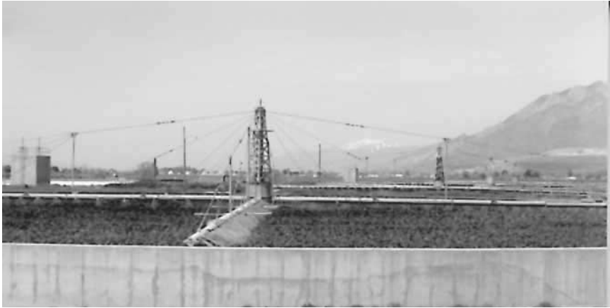
Figure 2.55 An intermediate-rate trickling filter.
