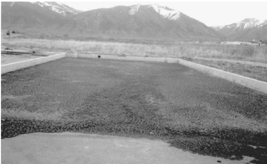
Figure 5.55 Photograph of a standard paved drying bed.
