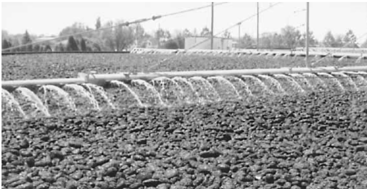
Figure 2.58 Rotary wastewater distribution system.
