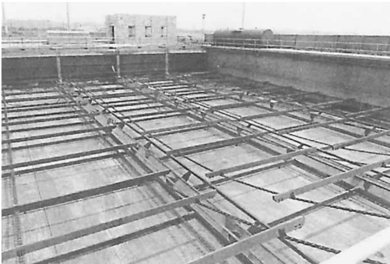
Figure 2.24 (a) Schematic diagram of a chain-and-flight rectangular clarifier tank. (b) Photograph of a chain-and-flight sludge-removal system.
