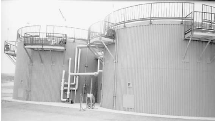
Figure 3.59 An autothermal aerobic digestion system.
