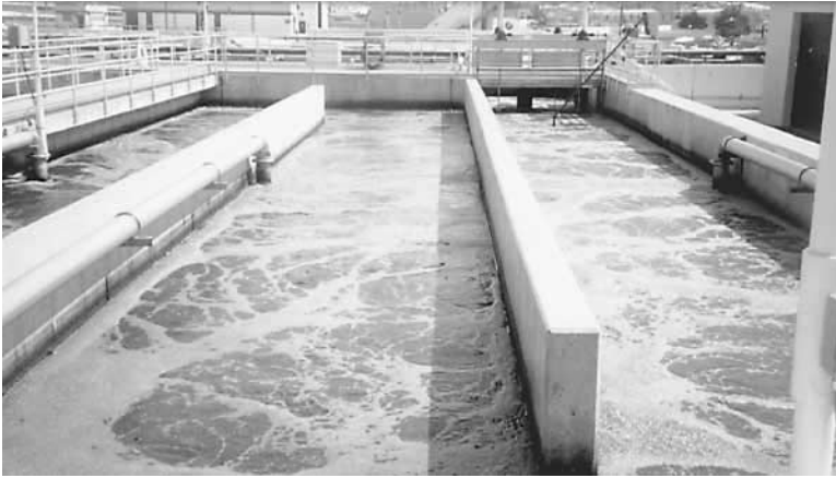
Figure 2.33 (a) Schematic diagram of a conventional plug flow activated-sludge system. (b) Plug flow activated-sludge system.
