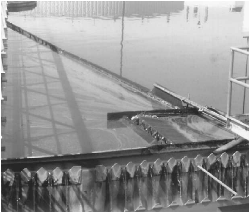
Figure 5.64 Scum-removal arm used in clarifier design.
