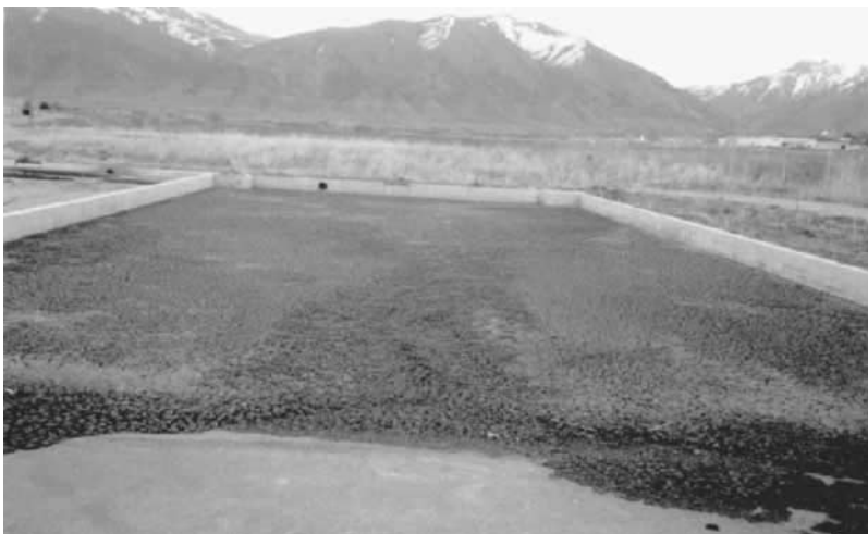
Figure 2.6 A biosolids/sludge drying bed.
