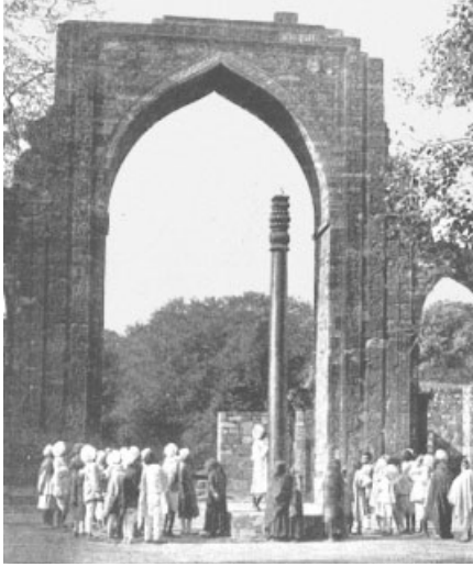
Figure 8.9 The forged Kutub iron pillar in Delhi. The pillar is shown to the right in the picture. (Reprinted from R. Hadfield, Journal of the Iron and Steel Institute , 1912, 85.)
