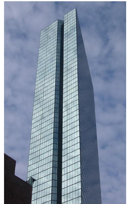
c / The John Hancock Tower in Boston vibrates naturally at a frequency of 0.14 Hz. Surprisingly, this frequency is the same regardless of the amplitude of the vibrations
