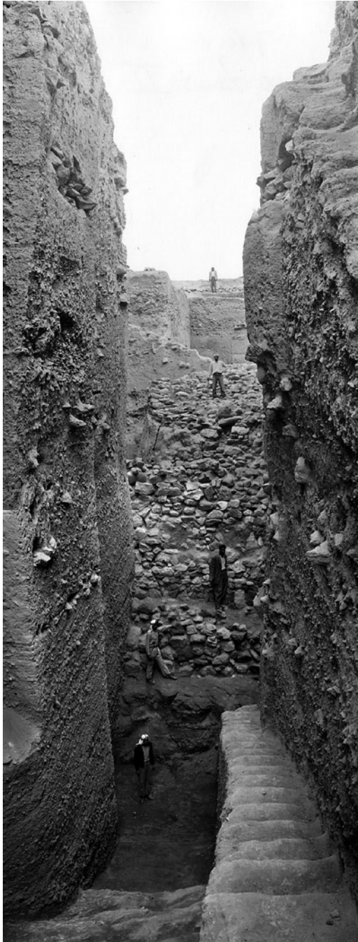
Jericho, the earliest known walled settlement by far. A view of the free-standing stone wall and moat, dated to the eighth millennium BC
