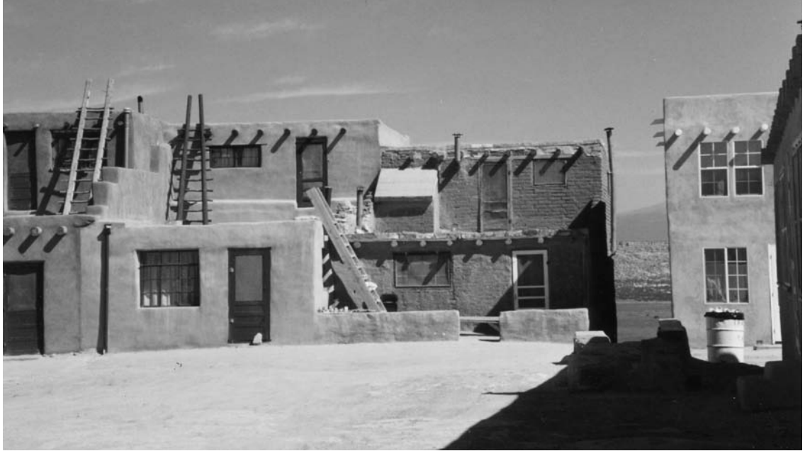
This photo shows a portion of an adobe house block at Acoma Pueblo in New Mexico. The architecture combines indigenous design with techniques brought by the Spanish—mud bricks smoothed with a mud plaster.
