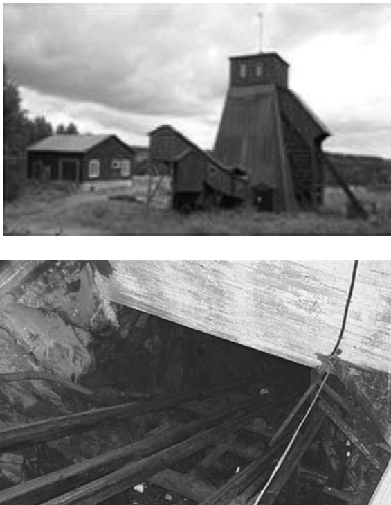
FIGURE 27.5 Storgruvan in Pershyttan, above and below ground.
