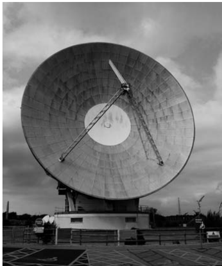
Figure 8.43 First dish antenna called ‘Arthur’ commissioned at Goonhilly Earth station (Courtesy: Madzany)
