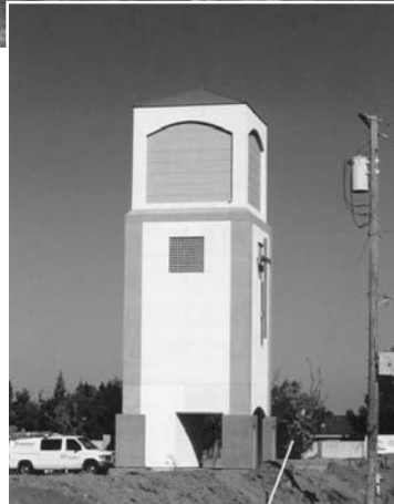
An interesting compromise. A free-standing church steeple? Actually, it's a relay tower for wireless communications, its design dictated by the fact that the property of a church was the best area to receive and transmit signals. The tower was modeled on a church steeple to conform it with the theme of the property. A similar concept is found in Cayce's readings for past Atlantis. Are we going too far? (Author's collection)
