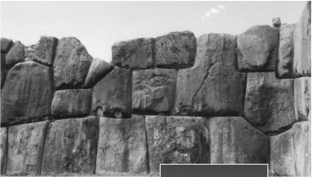
Sacsahuaman. Note the detail in just one short section of the wall. (Courtesy Judith Marx)
