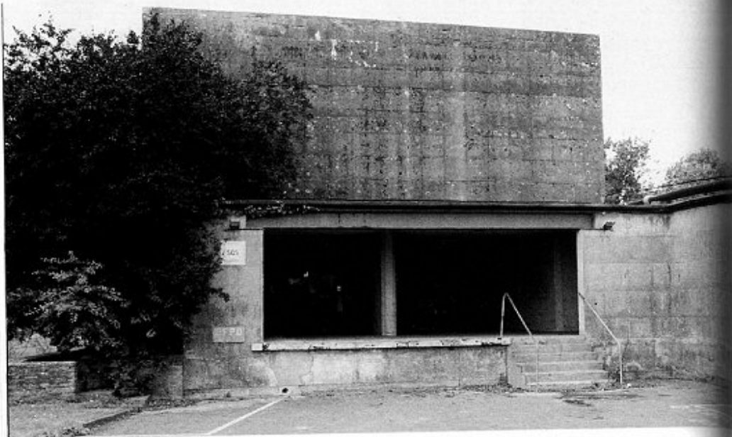
40. One of the nine heavily protected lift-shaft buildings at Spring Quarry.
