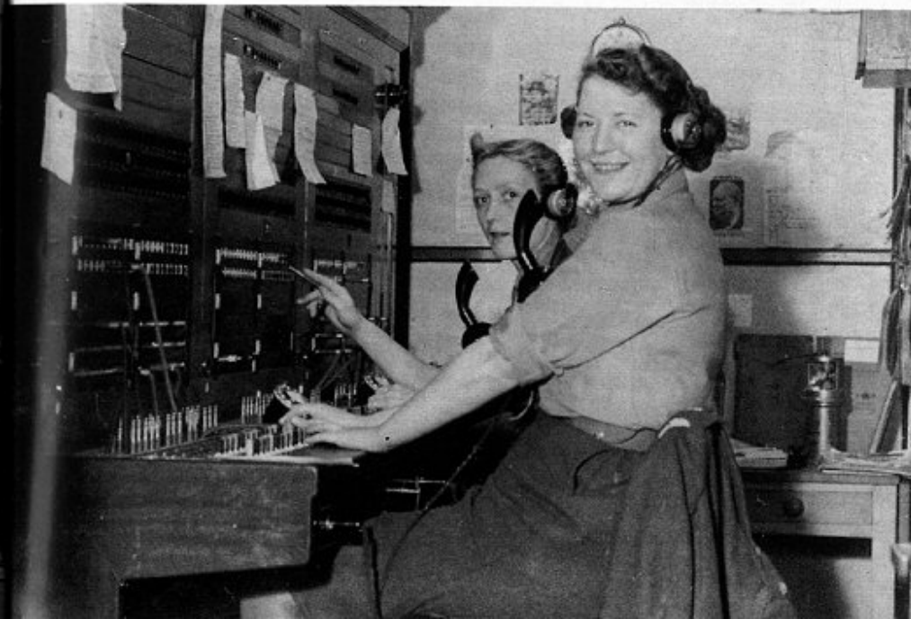
10. ATS Corporal Edna Bullen operating the underground private branch exchange at Tunnel Quarry in 1943.
