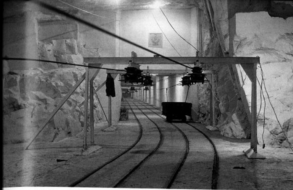
5. A superb view of Hudswell drift as seen from the lift bottom just after completion in 1938.
