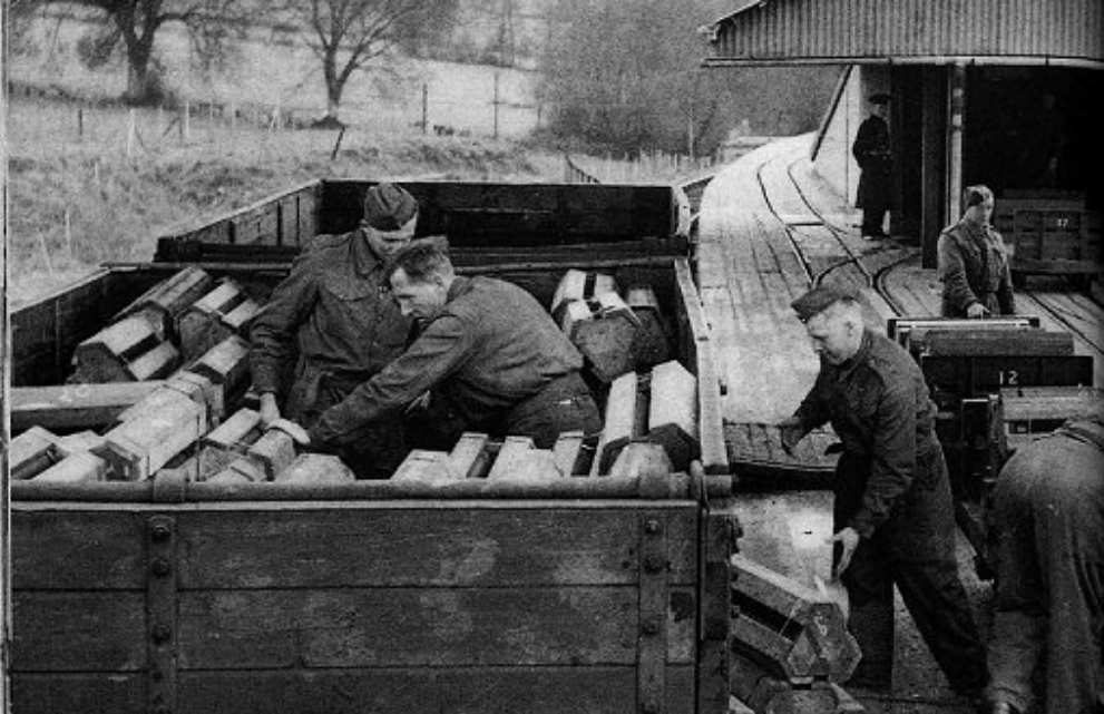
22. Unloading 155mm propellant charges at Farleigh Down in the autumn of 1943. Virtually all movements were now done via the tunnel belt and the aerial ropeway saw only intermittent use. Note the trucks adapted with end plates for work on the tram-creeper.
