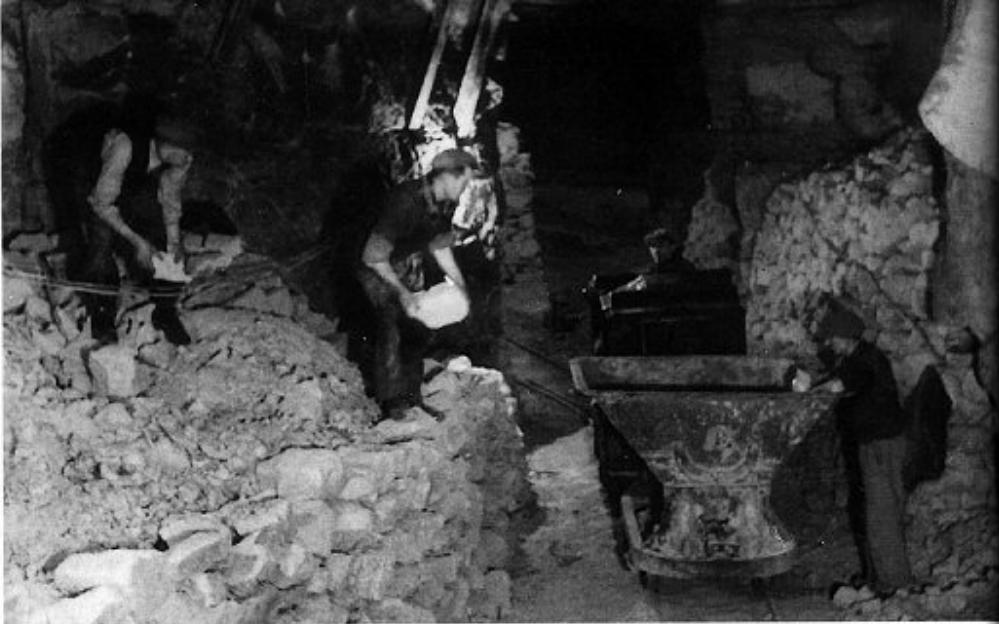
3. A diminutive Ruston diesel locomotive and Hudson tipper used to remove debris from the old workings. Virtually all the loading was done by hand following an unsuccessful attempt to use electrically powered mechanical excavators.
