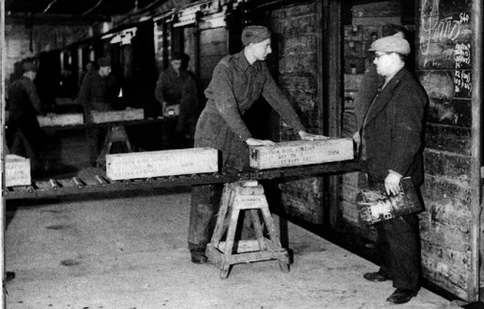
14. A large issue of anti-tank mine fuses being entrained from the south face of the underground loading platform at Tunnel Quarry in 1943. The portable gravity runways are linked to the belt conveyor on the platform.
