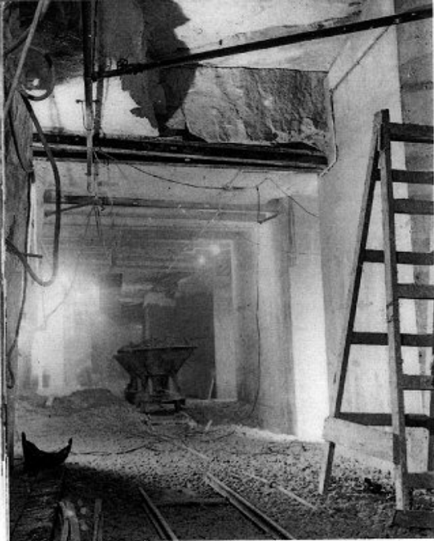
26. Construction nears completion at Eastlays. Floors are being graded with small stones prior to rolling and tarmac laying. Note the temporary cables festooning the walls.
