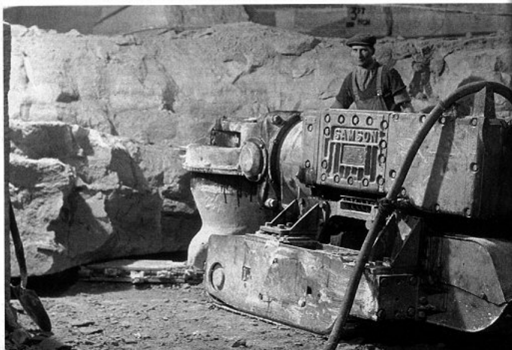
4. A Samson coal cutter at work in Tunnel Quarry in 1936. Note the rotating head slewed horizontally to undercut a large stone block.
