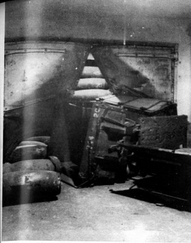
26. Construction nears completion at Eastlays. Floors are being graded with small stones prior to rolling and tarmac laying. Note the temporary cables festooning the walls.
