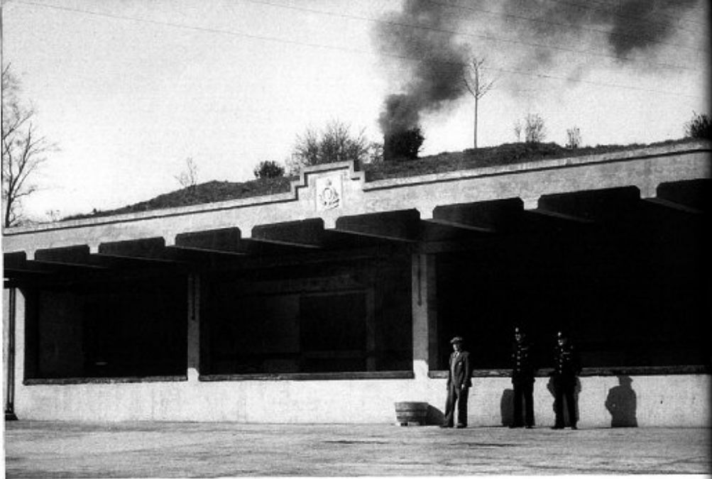
7. Tunnel Quarry Main Surface Loading Platform. Smoke in the background is from the boilerhouse chimney, which is directly behind the MSLP.
