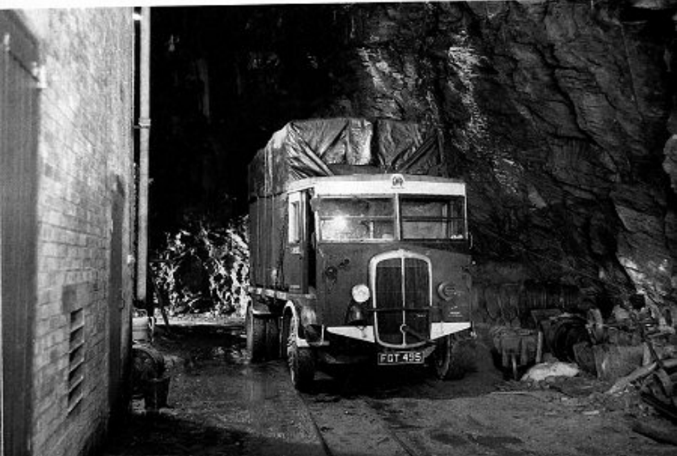
45. Manod Quarry. Inside the main entrance tunnel leading to the underground repository. The brick building to the left houses the power station and switch-room, 2 September, 1941.
