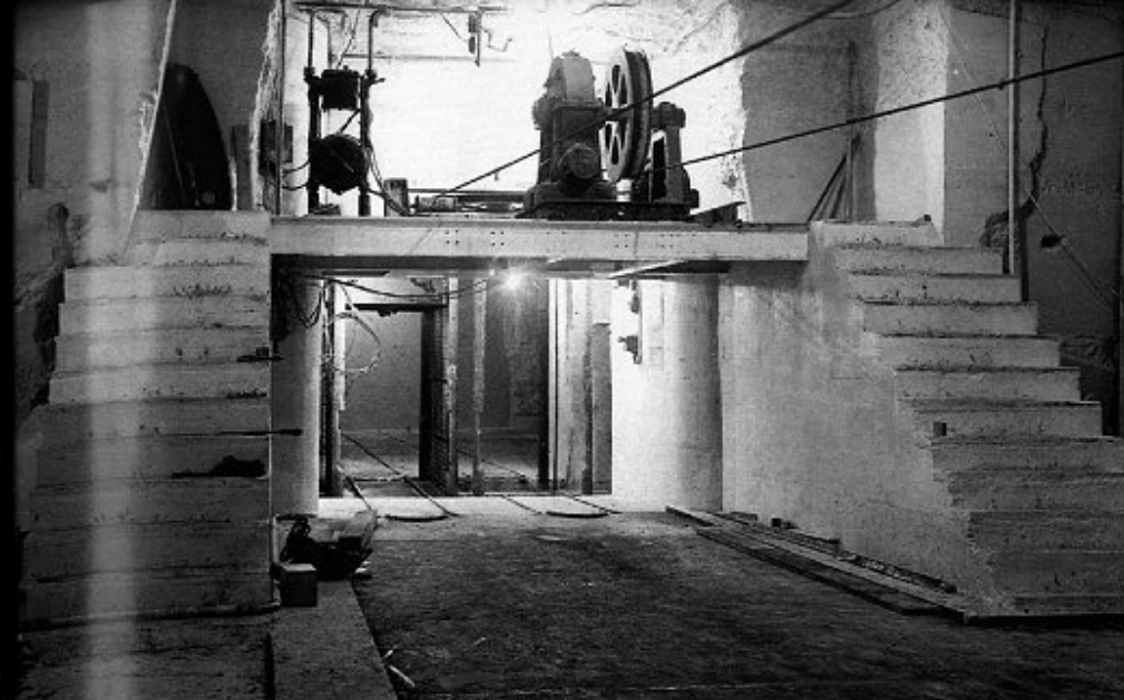
16. Hudswell North lifts nearing completion, with the temporary cages in use. The left-hand cage can be seen on the lower landing. This view, taken from the drift, shows the winding motor for the overhead rope-haulage working the drift behind the camera position. Tracks in the background serve Districts 8 & 9.
