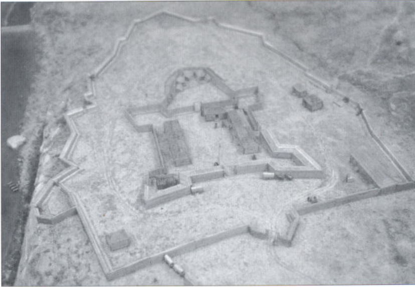
Model of Fort Ligonier, which Pennsylvania volunteers began building on Forbes' Road in 1758; in matters of basic design European military engineers made no concessions to the wilderness setting. Fort Ligonier consisted of a bastioned fort of earth and logs with an outer retrenchment of three and a half acres surrounded by a log wall. It was raided twice by the French during the fall, but served as the staging point for up to 6,200 British and American troops. (Fort Ligonier Museum)
