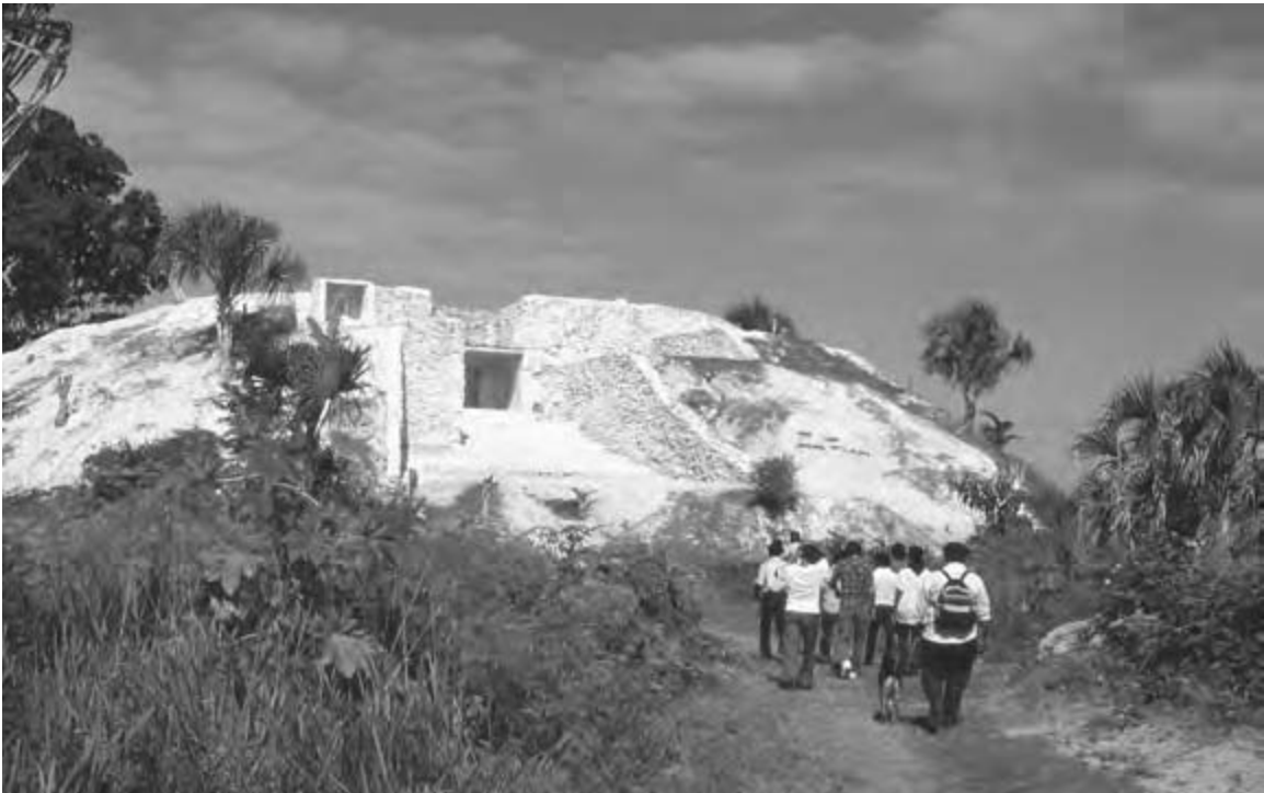
Classic building at Santa Rita Corozal, northern Belize, after excavation and reconstruction by Diane and Arlen Chase (Courtesy H. McKillop)
