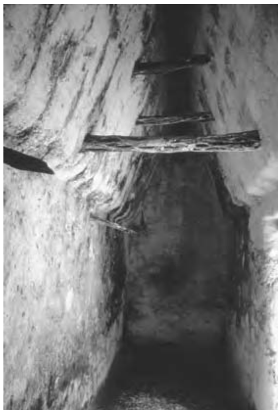
Above: Corbelled vault room construction in uppermost building of the Castillo at Xunantunich, Belize (Courtesy H. McKillop)
