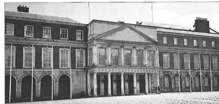
The State Apartments, Dublin Castle. It was here, during a meeting about the best way to suppress the Irish Volunteers, that the Government became painfully aware of the Rising, as members of the Citizen Army launched an abortive attempt on the castle gates. (Courtesy David Murphy)
