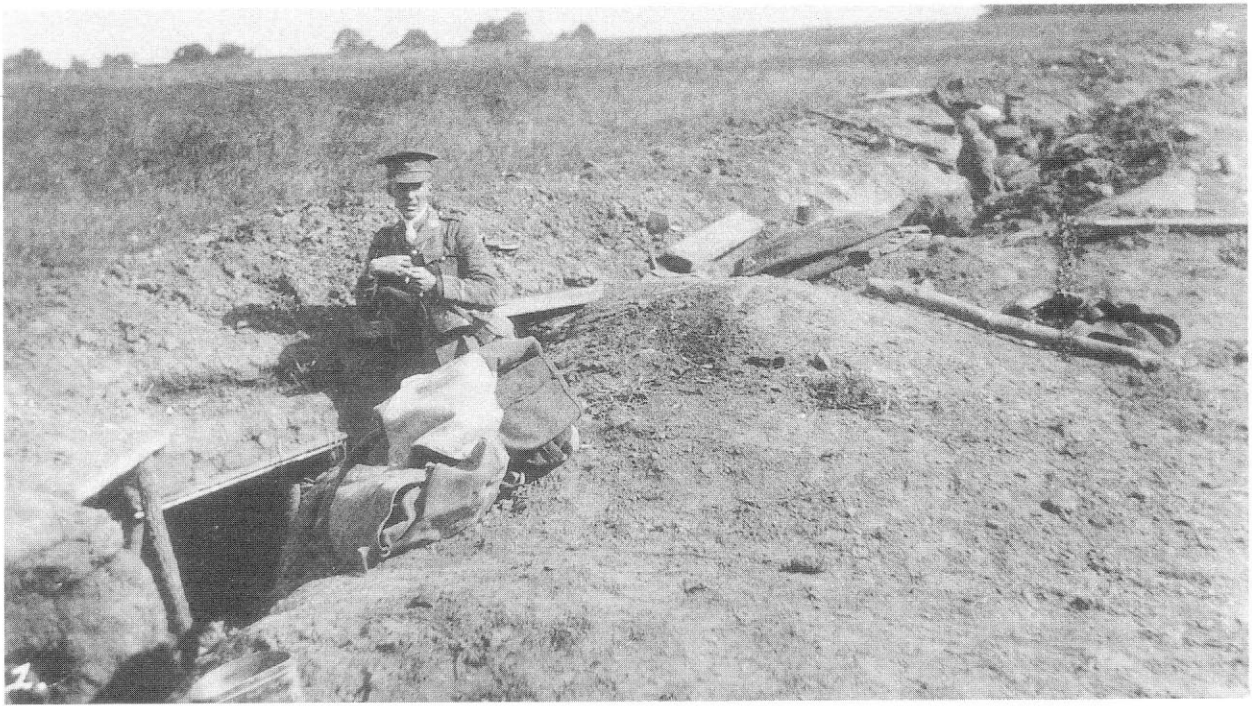
Type of shallow front-line trench at the beginnings of trench warfare on the Aisne, 22 September 1914, manned by 1/King's Own, 4th Division. Note rudimentary parapet and dug-out entrance left of the officer. (Cameronians Museum)
