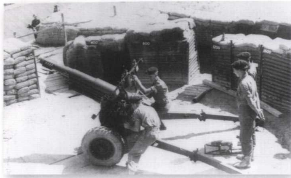
ABOVE LEFT Royal Marine gunners in a forward base take post, ready for a fire mission. The 105mm pack howitzer gun pit has been constructed from sandbags, corrugated galvanized iron and six-foot pickets. The bearings (in milliradians) can be seen painted around the pit. It was essential to build up such emplacements rather than dig down, as heavy rain could easily flood a position. (RM Museum)
