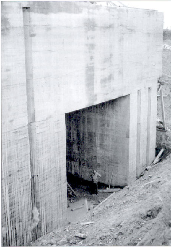
The Sottevast missile bunker near Cherbourg was configured like the Watten bunker, but using construction techniques to minimize the risk of Allied air attacks. Only this section was completed by the time the area was captured by the US Army in June 1944 after the Normandy landings. (NARA)
