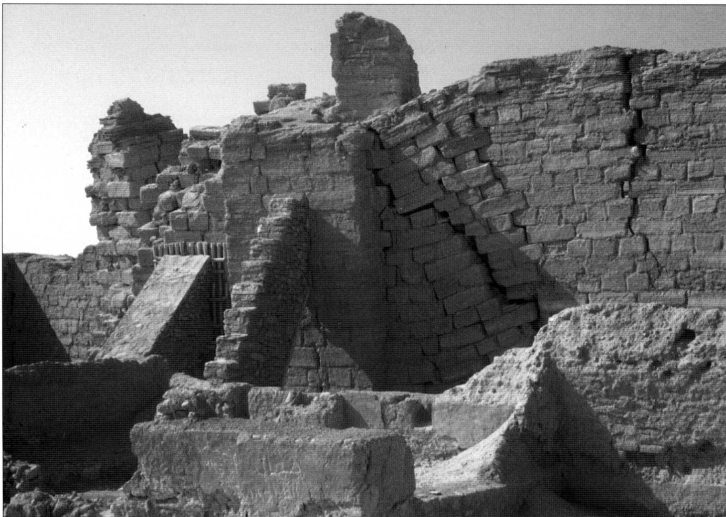
Tower 14 at Dura Europos, viewed from within the town. The Persian attackers successfully undermined the four walls causing the tower to come apart, thus preventing its use as a platform for catapults and archers. The buttress is a modern addition. (© M. C. Bishop)
