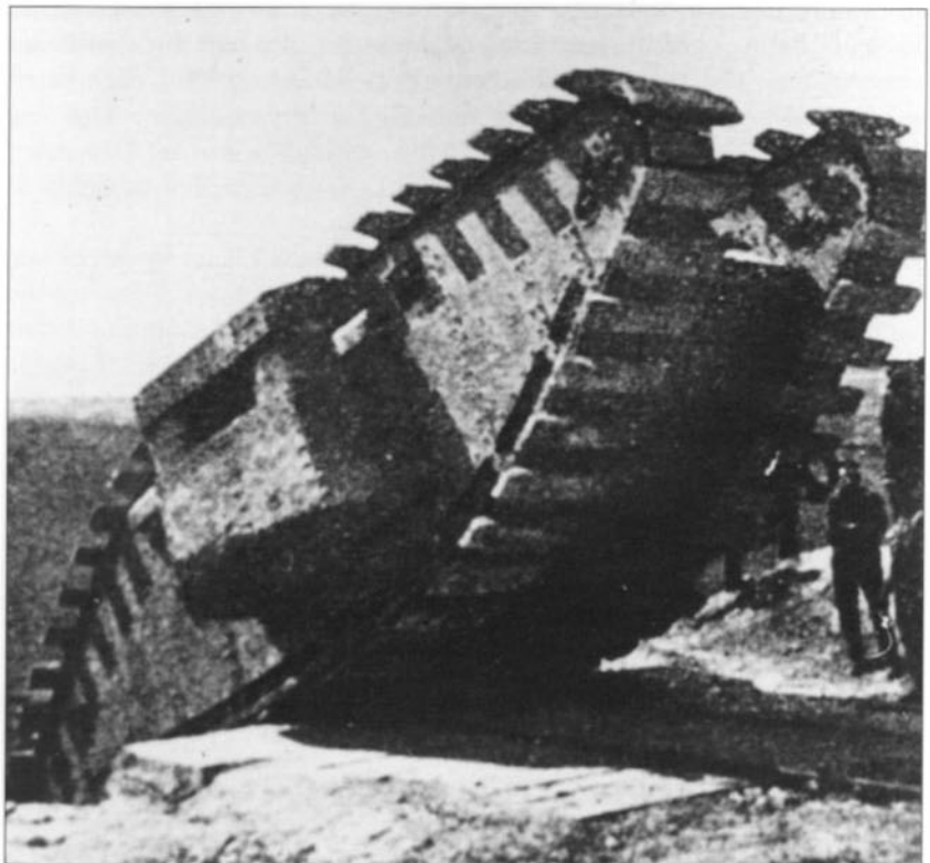
A poor but rare photo of a Female tank, fitted with special climbing spuds, tackling a mock sea wall during training for Operation Hush. This climb must have been a driver's nightmare. Had the operation gone ahead Mark IV tanks would have been employed.
