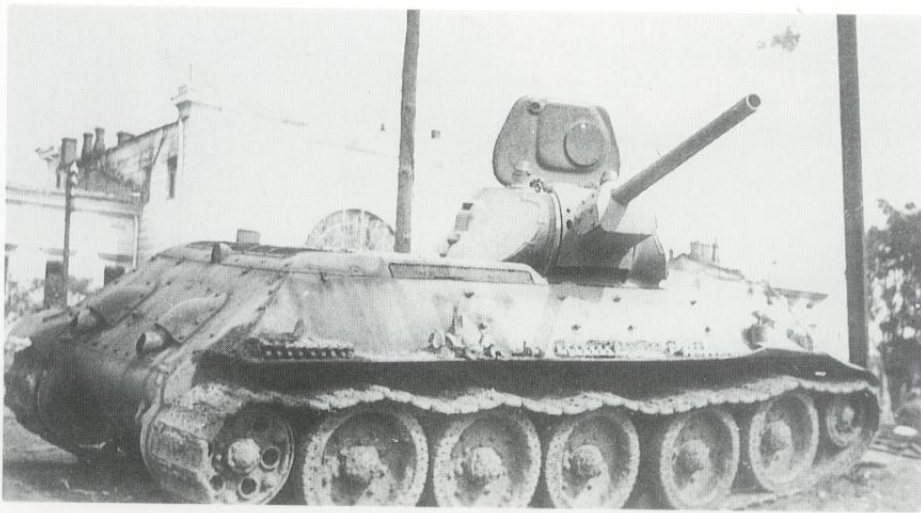
A T-34 Model 1940 abandoned at Vinnitsa in western Ukraine following the Dubno-Brody tank battles at the end of June 1941. Small numbers of T-34s survived these battles, but many were abandoned due to breakdowns and lack of spare parts.
