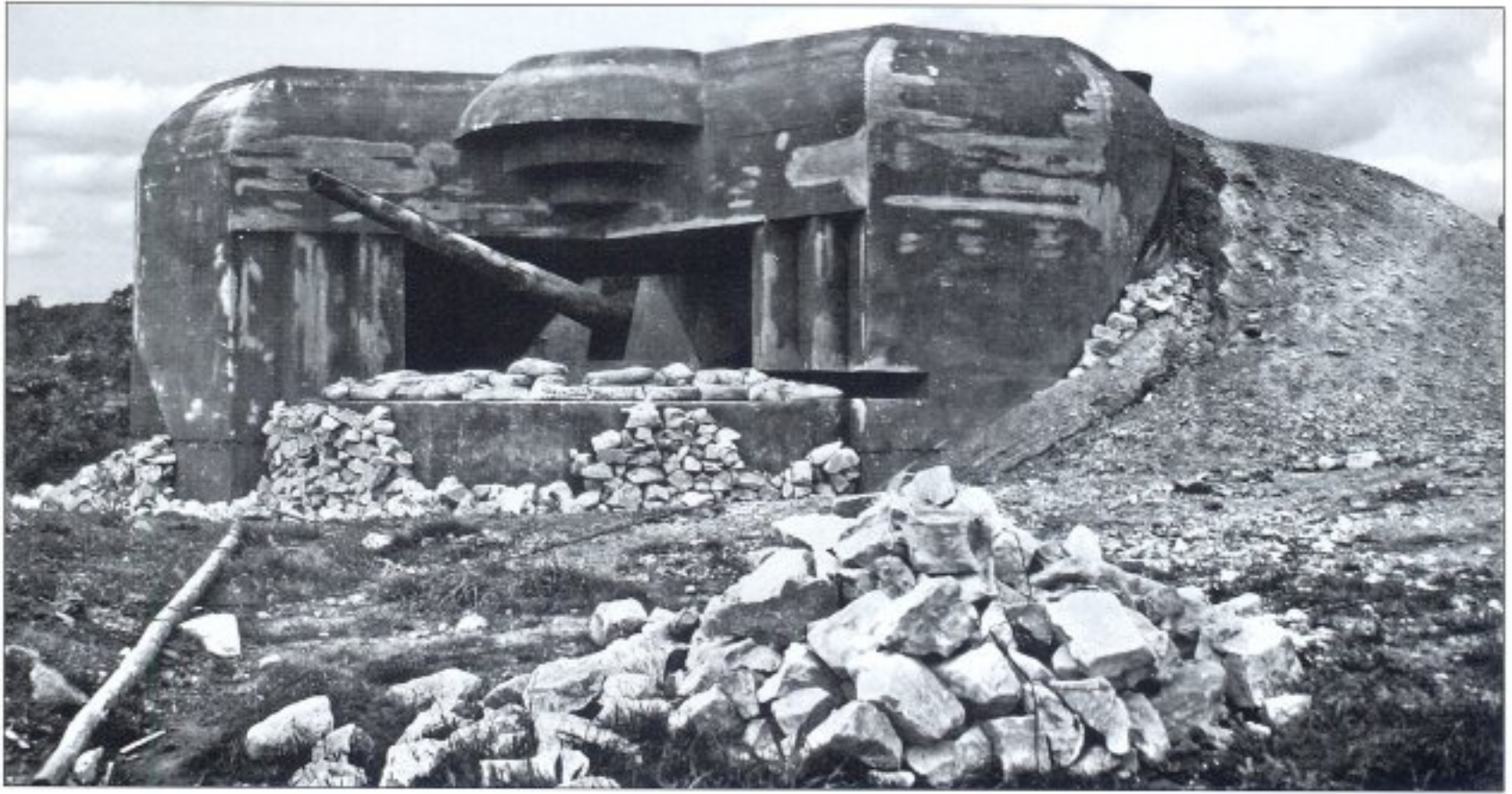
This Rheinmetall 150mm SKC/28 in a coastal C/36 mount with non-standard gun-shield was one of four guns of MKB Landemer, 6./MAA 260, positioned in an M272 casemate, part of StP 230 in Castel-Vendon to the west of Cherbourg. (NARA)
