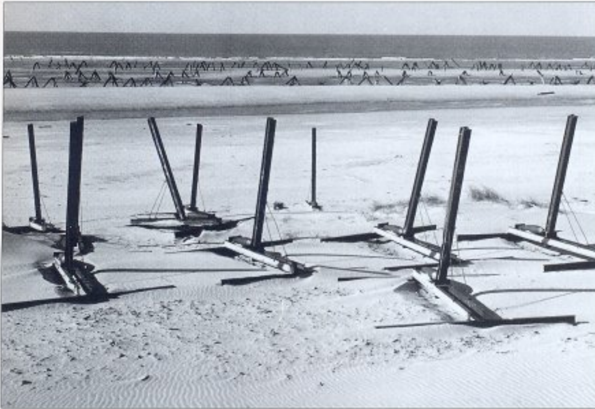
A fairly typical example of beach obstacles in the Fifteenth Army sector east of Dunkirk in September 1944. The obstacles in the foreground are Nussknacker (nutcrackers) made from French artillery projectiles with a pivoting steel trigger designed to blow up under landing craft or tanks. Closer to the sea are a variety of obstacles, mainly wooden tetrahedrons but also some steel Czech hedgehogs. (NAC P-174349 Ken Bell)
