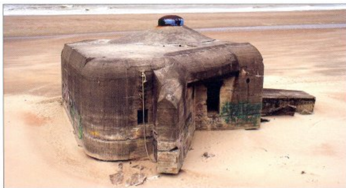
Coastal erosion has left many bunkers stranded on the beach, like this H120 artillery observation bunker on Platier d'Oye east of Calais. It is an interesting example since it is still fitted with its 27P01 armored cupola, a feature that was removed from most bunkers after the war due to its scrap value. (Author's collection)
