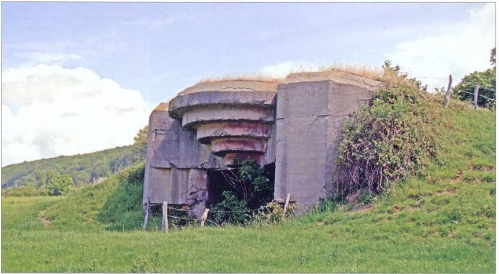
This is one of four M272 casemates of MKB Vasouy, 9./MAA.266, opposite Le Havre which was armed with a 150mm Tbsts.KL/45 . (Author's collection)
