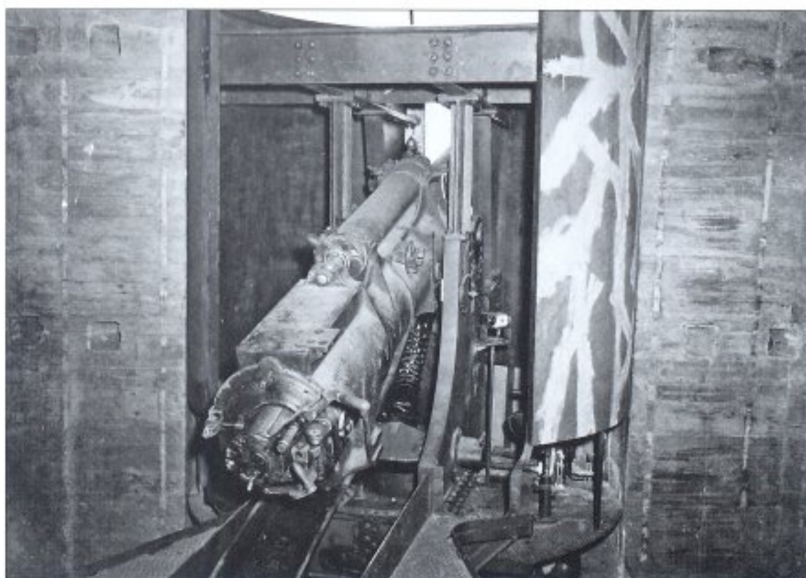
The St. Chamond 155mm K420(f) gun was adapted for coastal defense with a special armored mount to fully enclose the embrasure. This example is mounted in an H679 casemate of MKB Gatteville of 7./HKAR.1261 near Cherbourg. (NARA)
