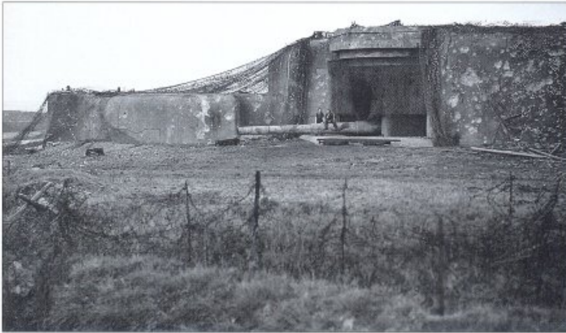
This is Bruno, one of three gun casemates of MKB Friedrich August of 2./MAA.240 in La Trésorerie, armed with a massive 305mm SKL/50 gun. It was captured by the Canadian North Shore Regiment during Operation Wellhit . (NAC PA-174409 Donald Grant)
