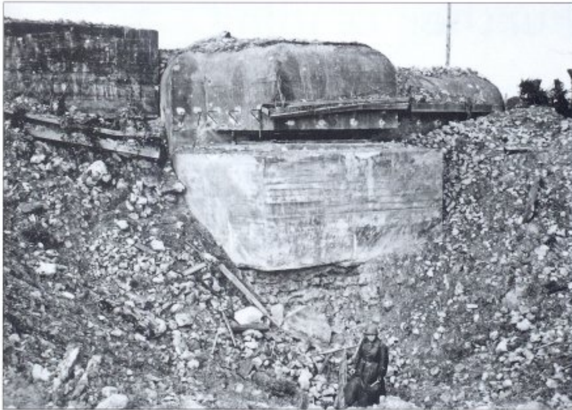
MKB St. Marcouf engaged in duels with Allied warships on D-Day and the site was heavily bombed and shelled. This massive crater in front of its observation post gives some idea of the intensity of the fire. (NARA)
