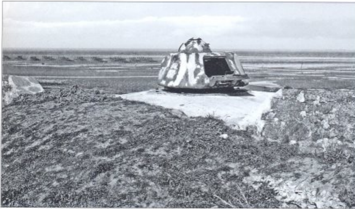
Tobruks were also used to form the basis for Panzerstellungen using surplus tank turrets like this French APX-R turret with 37mm gun being used in the strongpoint at St. Marcouf-les-Gougins on the Cotentin coast north of Utah Beach. (NARA)
