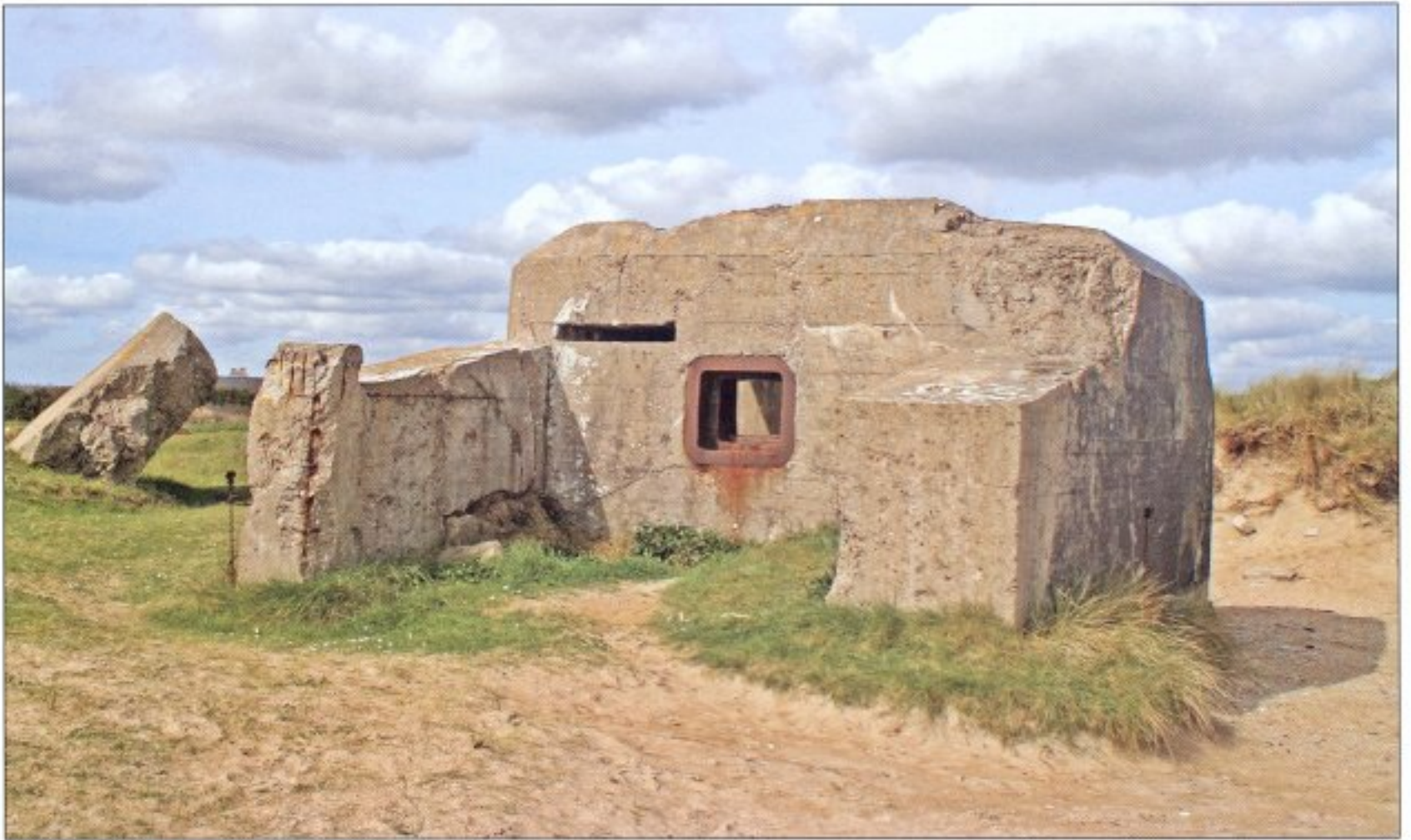
A fairly typical example of an enfilade casemate for a Skoda 47mm Festungpak 36(t), one of two located on the right flank of strongpoint WN10 to the north of Utah Beach on the Cotentin Peninsula. The metal enclosure for the ball mount is still present, though the gun itself has long since been scrapped. (Author's collection)
