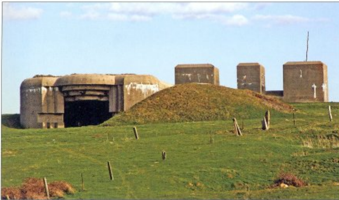
Stützpunkt 164, between Cap Gris-Nez and Cran aux Ouefs, was the site of MKB Tilly of S./MAA.244 with two M270 casemates armed with 150mm guns. The three large pillars near the casemate are the V143 base for a massive Mammuth surveillance radar that supported the neighboring Batterie Todt and other heavy gun batteries in the area. (Author's collection)
