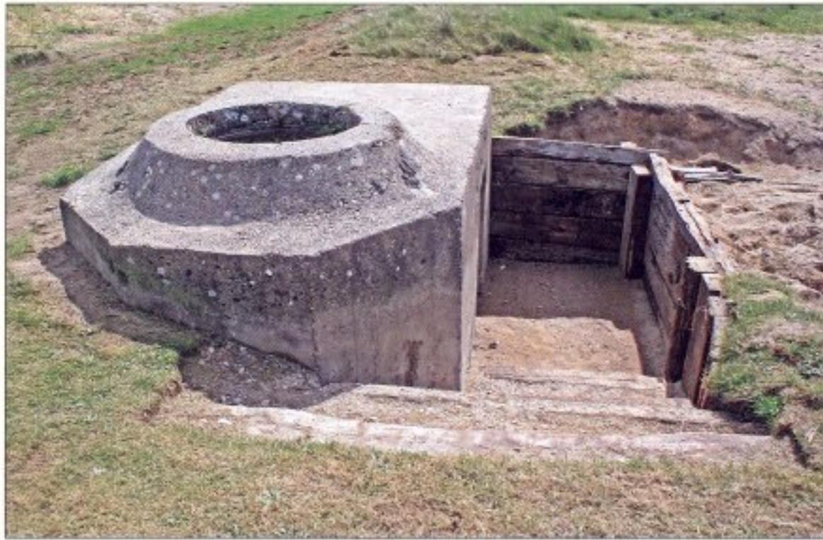
Tobruks were generally buried since their protection was only B1 standards, 1.5m thick or less. Usually the tobruk included a small room for ammunition storage and crew shelter, which was usually accessed through a small door, requiring an adjacent trench. (Author's collection)
