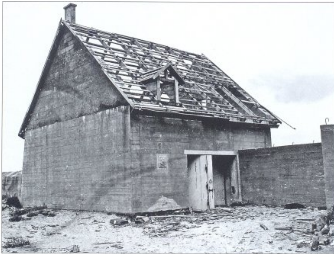
This 75mm enfilade casemate on the Cotentin coast north of Utah Beach has been camouflaged to resemble a house by erecting a false roof over the structure. This particular casemate was built into an anti-tank wall built to prevent easy access off the relatively flat beach, a common type of obstacle on the Atlantic Wall. (NARA)
