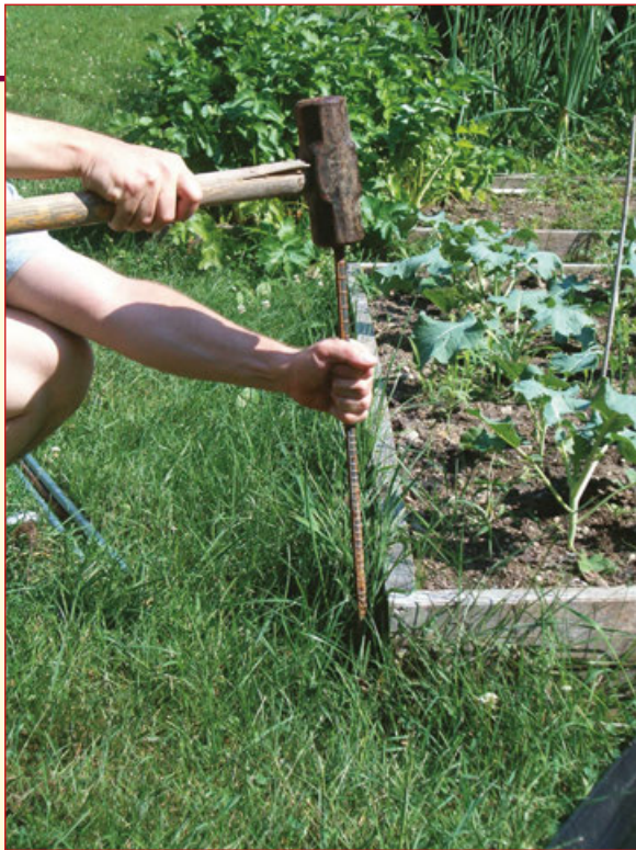
➤ Driving the rebar into the ground.
