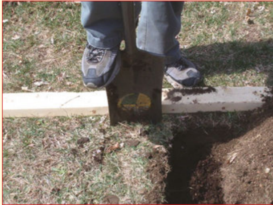
⌘ Digging the second trench. Beware the author's stylish footwear!
