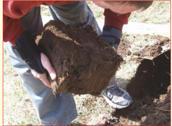
⌘ Putting spits in the trench upside down.
