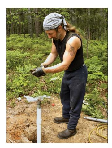
Dropping a long, weighted string down the driven well pipe to test how far underwater a well point has penetrated.
