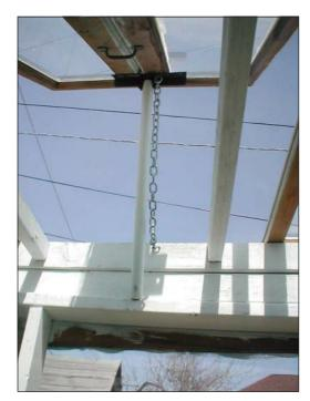
some reflecting fabric. Lastly, I think in the future, I will completely rebuild the roof, using the windows for a gable type structure. It will force me to use some sort of poly material to cover up the gable ends. The current pitch of the roof is not enough to slope water off the windows completely.
