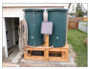
assembly from recycled wood, held together with new carriage bolts because the total weight of all the water when full is approximately 1700lbs. This frame is resting on eight 2"-thick, 18" square cement pads to prevent sinking. The barrels are raised to increase the head pressure and decrease the work load on the pump.
