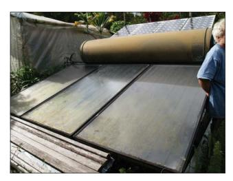
A solar water heater ("collector panel"). Radiated electromagnetic energy from the sun is absorbed by a black absorber panel, which heats the water in pipes connected to the panel.
