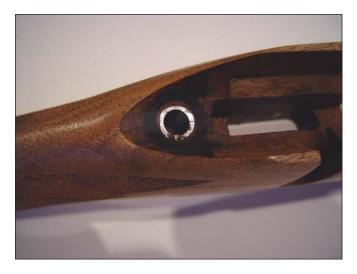
Pillar bedding sleeves are sometimes used to encourage a higher degree of accuracy in a hunting rifle.
