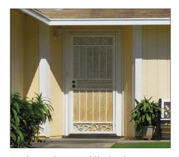
A steel security door over a solid hardwood core entry door is an adequate amount of door security for almost any neighborhood. Both doors must be properly hung to be completely effective, and must be installed with multiple locks and a reinforced jamb.
