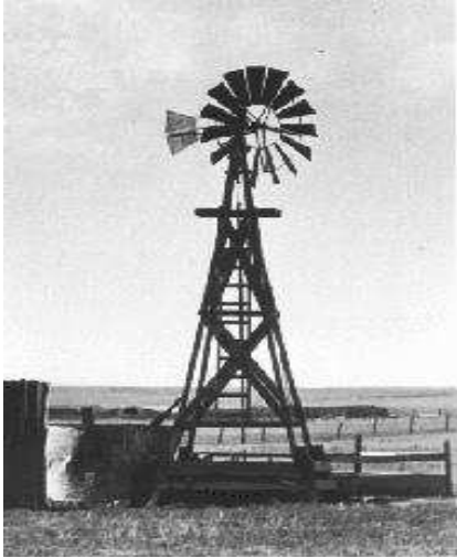
Figure 4 Horizontal Axis Wind Mill
