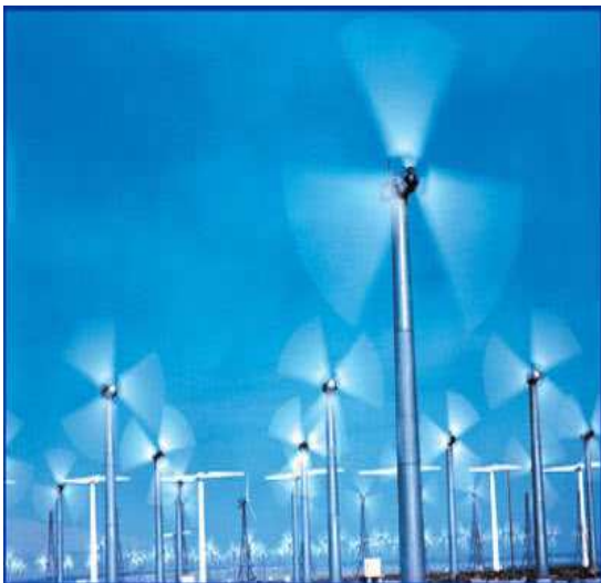
Figure 7 Wind Form Power Plant
