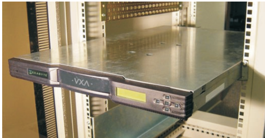
Figure 10. Placing the autoloader on the rails
