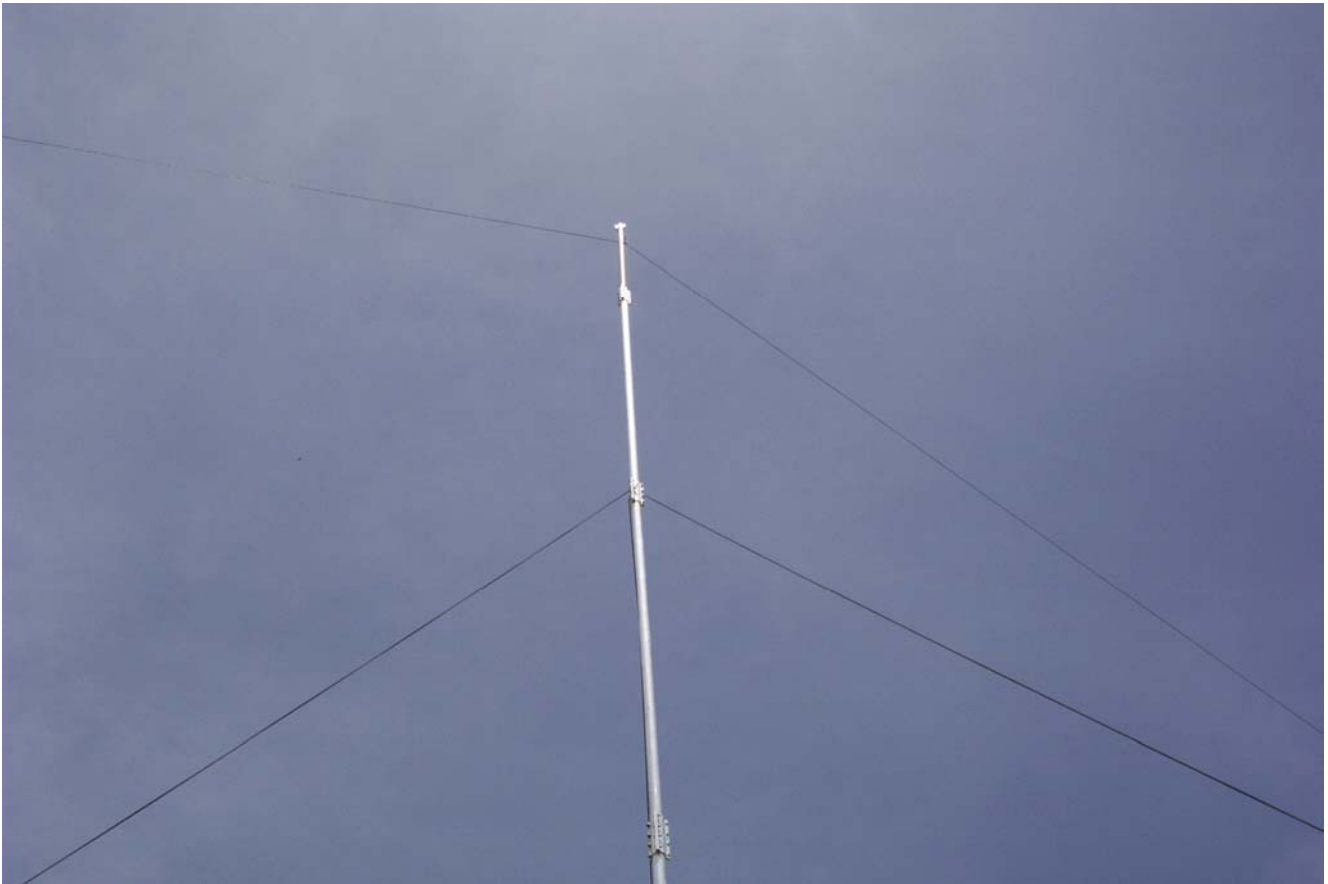
AS-WV-xxx Antenna supported at top with rope halyard. Top of mast is insulated model of mast is AS-PEN-38.5 and is 38.5 feet tall.
