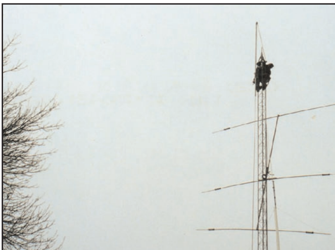
Hoisting the beam its last several feet to the top of the 62-foot tower, K6IMN gently moves the Mosley TA-33 into place.
