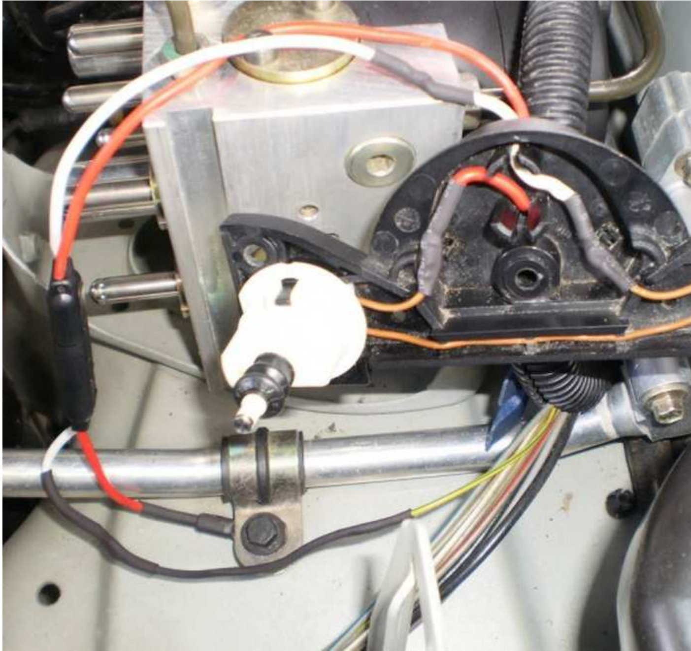
This is what it looks like plugged up.
