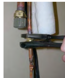
Installing the Line Set on the Indoor unit stubs
